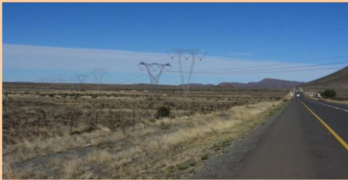
Plate 5: View of proposed powerline and the existing powerline crossing the main road.
