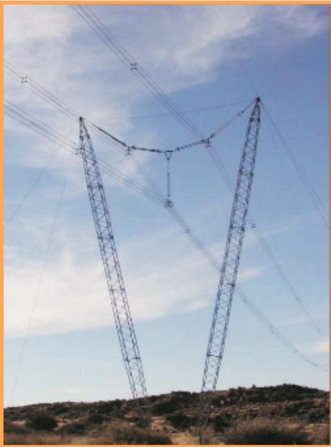
Plate 8: Compact cross rope suspension tower (Pallett, 2009)
