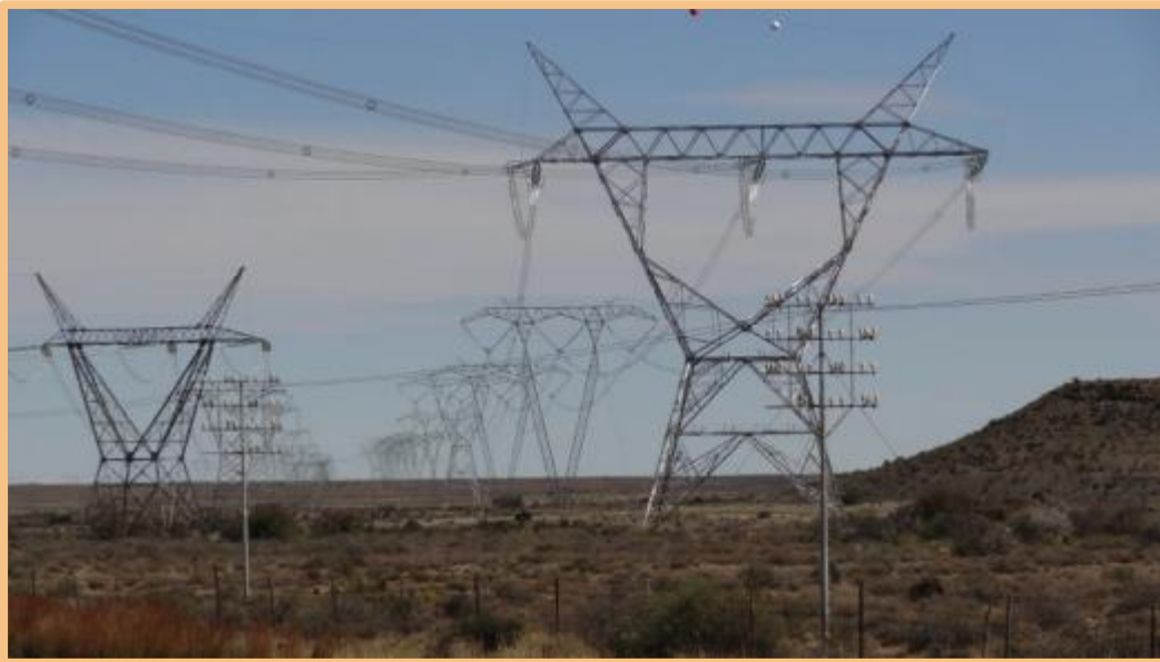
Plate 6: View of existing powerlines from a distance.
