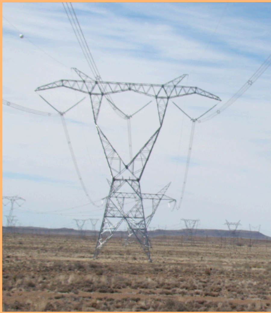
Plate 7:Self Supporting suspense tower (H. Mlotshwa, 2012)
