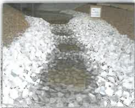
Figure 1 Example of a rock pitched chute directing water away. Retention areas in the chute slow water down. Swale
