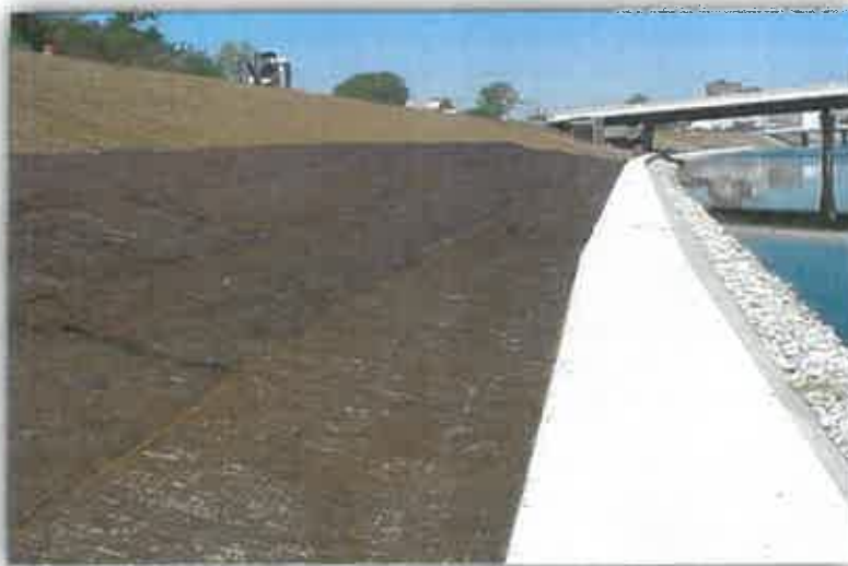
Figure 2 Geo-fabric installed and pegged down on a slope to retard soil erosion. Vegetation may grow through the blanket over time.
