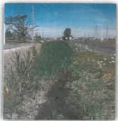
Typical application of a deflection berm to avoid erosion of a pipeline route
