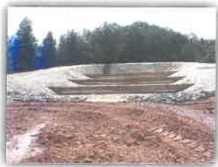
Figure 5 Multiple silt fences installed down a slope
