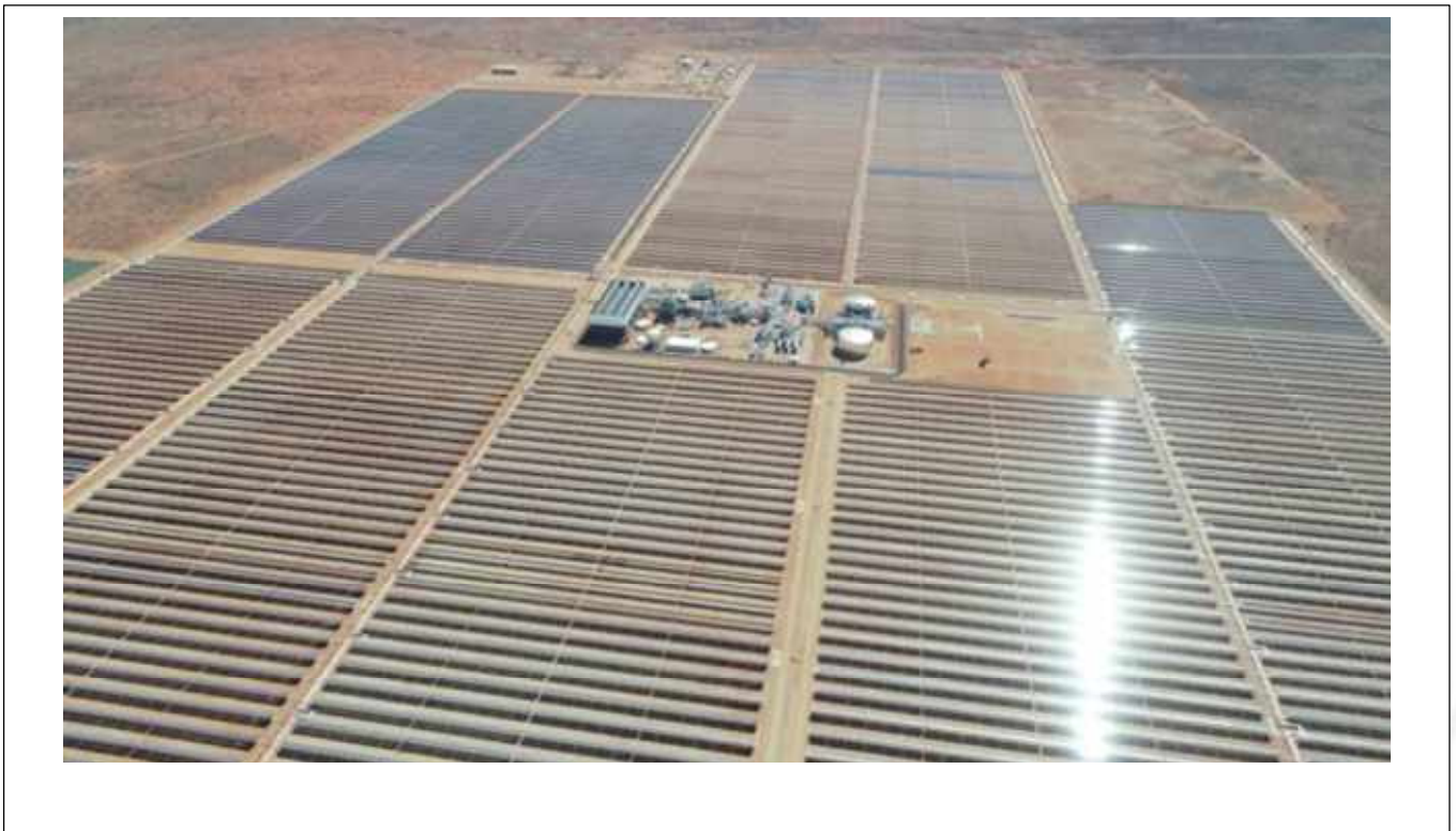
Figure 6.4: An aerial view of the operational Ilanga 1 CSP facility located in the north western corner of Lot 944 (source: https://www.ee.co.za/article/black-company-makes-renewable-energy-history.html ).
