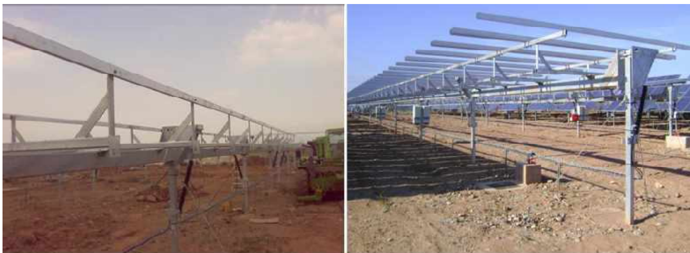
Figure 3.7: Frame, structural details (Photo courtesy of Igeteam, 2011).
