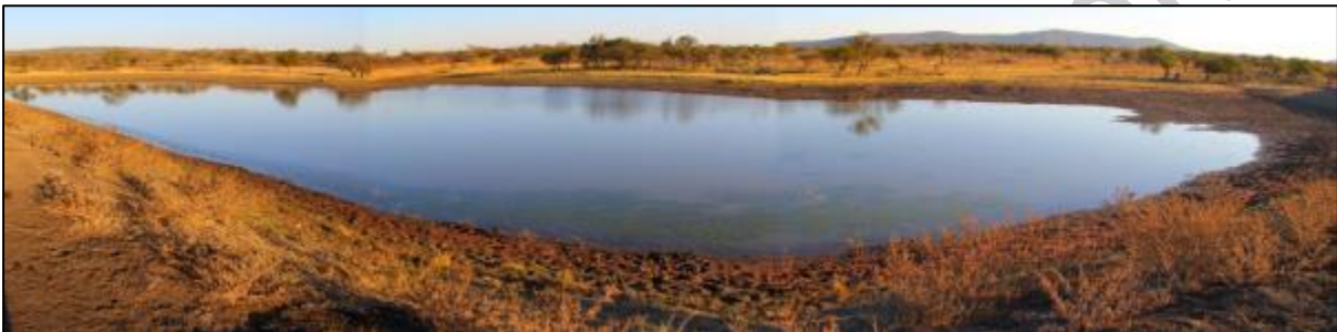
Figure 24: A view of Dam 5
