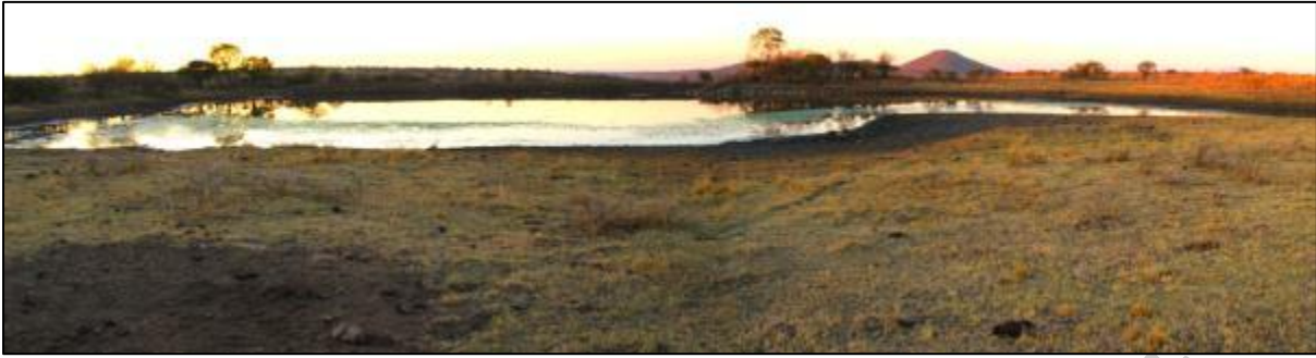
Figure 23: A view of Dam 4
