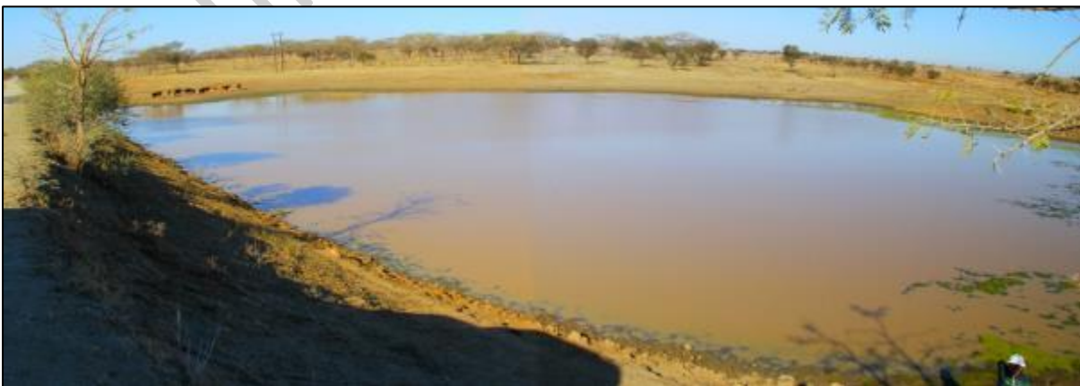
Figure 22: A view of Dam 2
