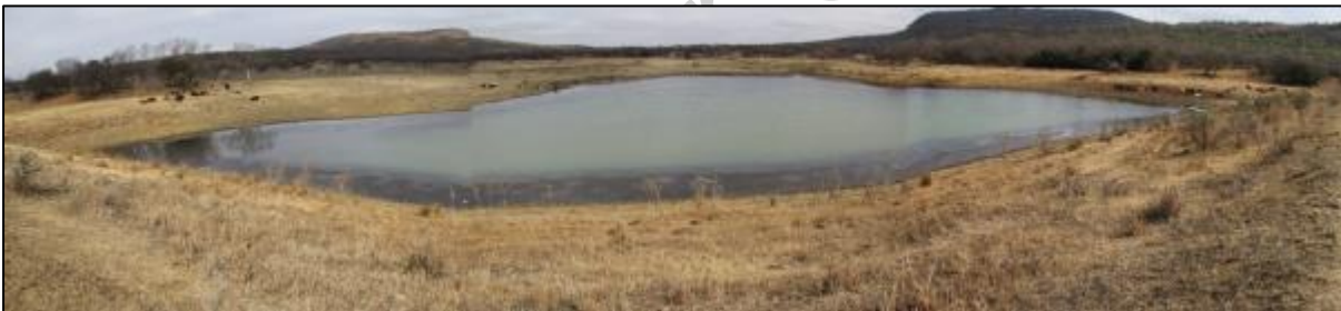
Figure 21: A view of Dam 1
