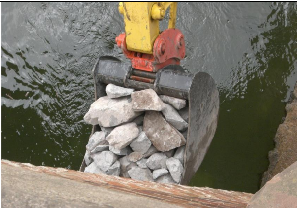
3. Place scour rock
