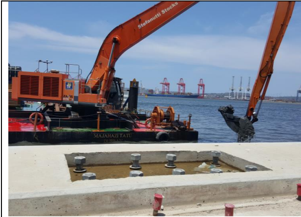
1. Dredge to required level
