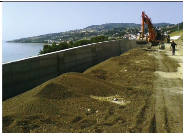
4. Backfill & install civil services
