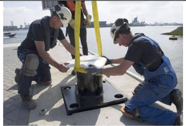
6. Pave & install quay furniture
