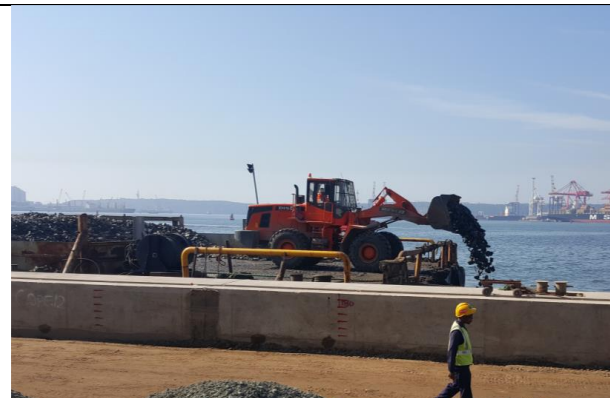
3. Place scour rock
