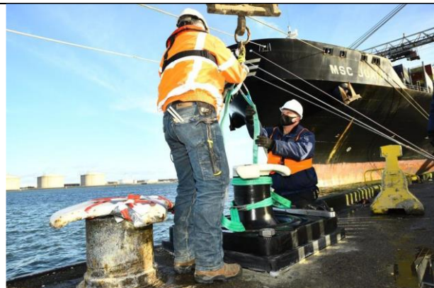
6. Install quay furniture
