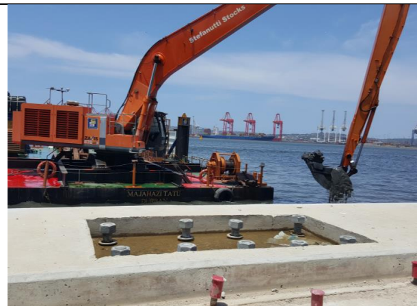
1. Dredge to required level
