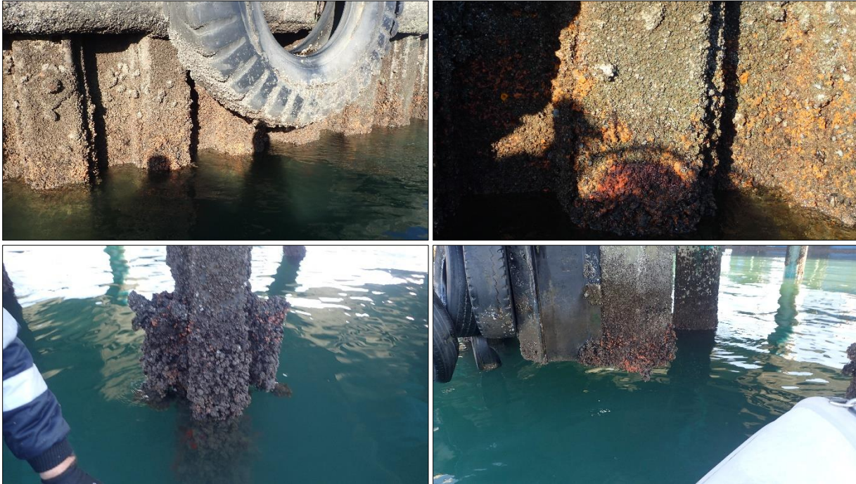
Figure 40: Photos showing encrusting organisms on the sheet pile quay wall at the Old Tug Jetty (top) and on piles near the Old Tug Jetty (bottom).
