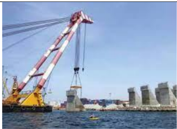
2. Place counterfort units & block work
