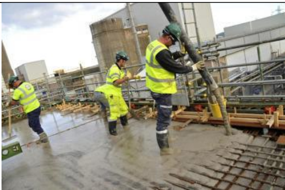
5. Install civil services & place stitching concrete
