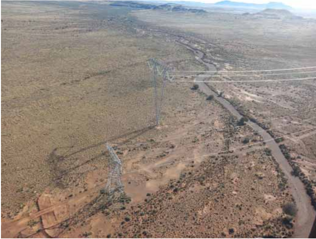
Plate 10: Pylons and access tracks in wide open floodplains near a main channel – exposed soils are at risk of surface wash and erosion, and stormwater management measures are important.
