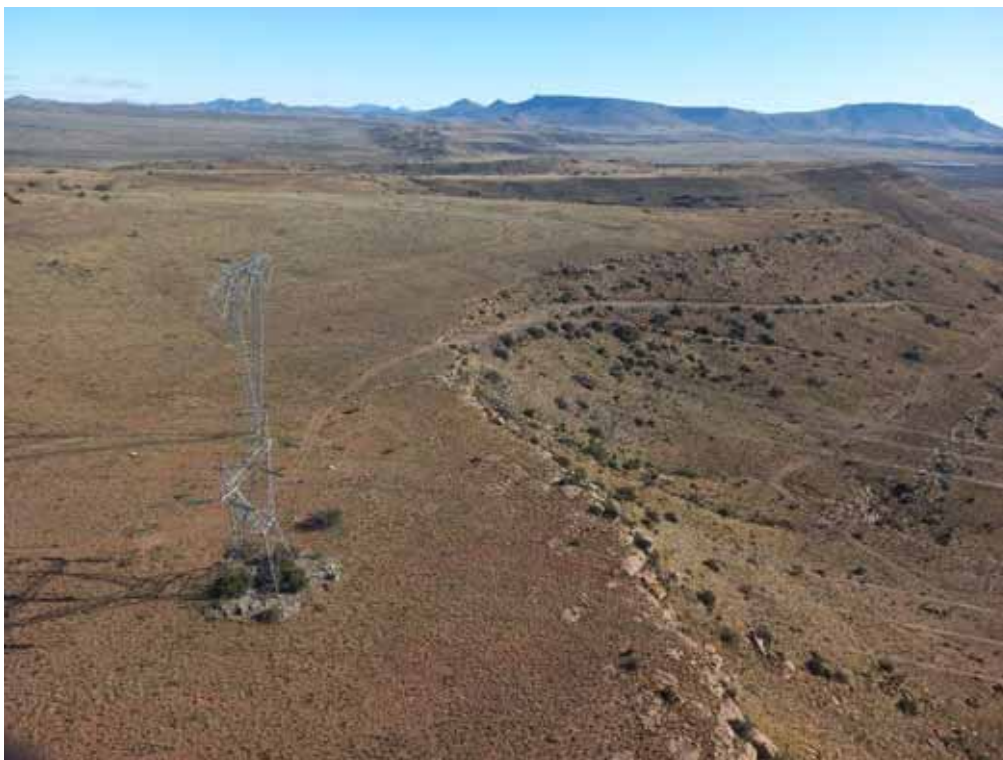
Plate 9: An existing pylon situated on a flat top, with an access track traversing a slope. The disturbance impact on soils seems to be limited to the pylon footprint and the access track with no obvious signs of erosion. The soils and rock in these areas are less prone to erosion, but care must be taken along access tracks to prevent channelized runoff and accelerated flow down slopes.
