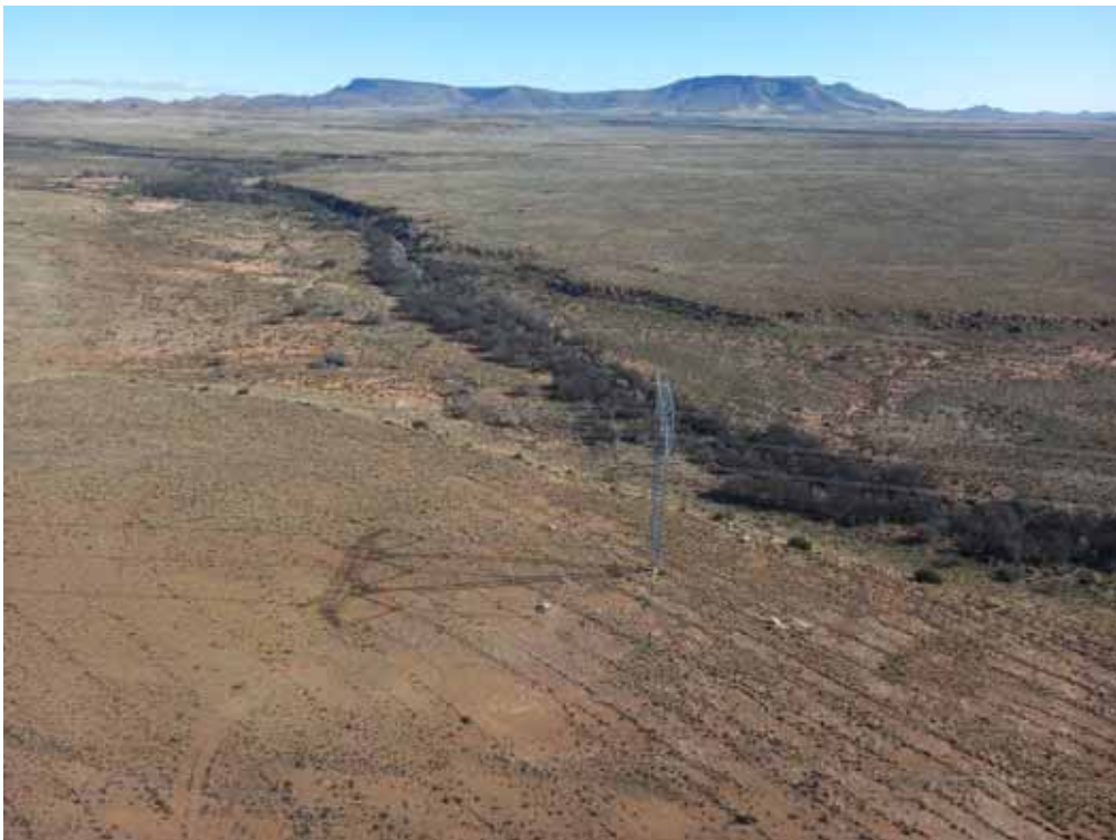
Plate 4: One of the existing gridlines on the eastern end of the Corridor, with a pylon placed to span the riparian area.
