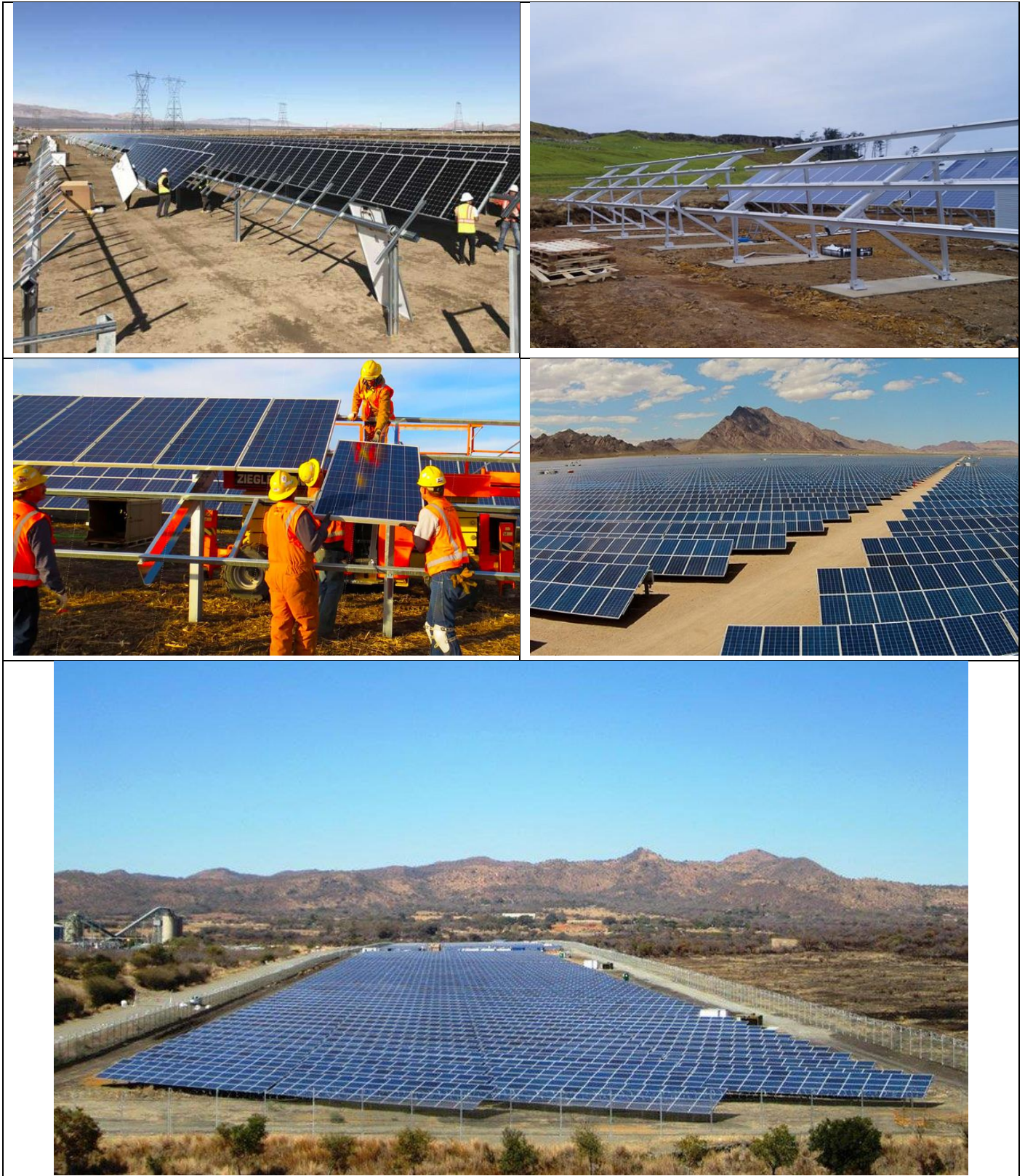
Figure 2.7: Photographs of the construction phase of a solar facility similar to the Highveld Solar PV Facility (Source: https://medium.com/@solar.dao/how-to-build-pv-solar-plant-6c9f6a01020f ; https://www.shutterstock.com/video/clip-1028794-workers-mounting-panels-on-solar-power-plant-construction ; https://www.esi-africa.com/renewable-energy/kenya-construction-solar-farm-gets-green-light/ )
