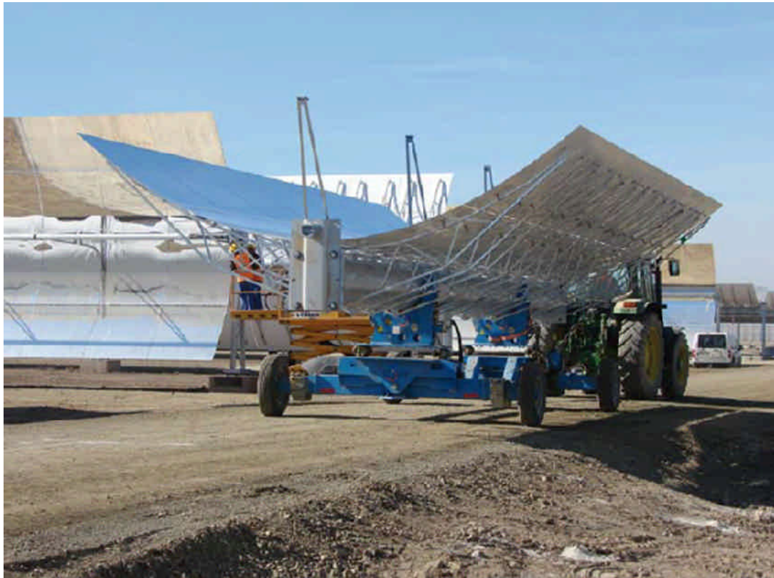
Figure 2.5: Photograph illustrating the transport of a built parabolic trough on the development site (Source: Siemens AG).
