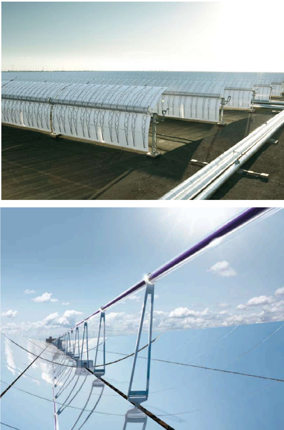
Figure 2.1: The bottom photograph illustrates the parabolic troughs together with the receiver tube (bottom photograph) and the pipes conveying the heat transfer fluid (top photograph) (Source: Siemens AG).
