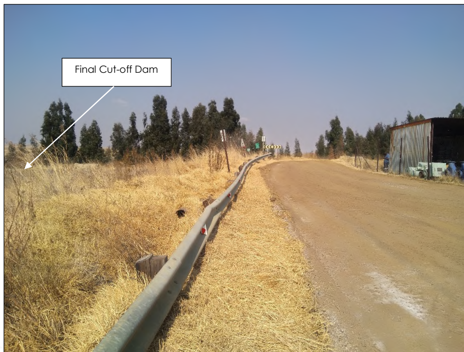
Figure 2.4: A view of the existing access road located adjacent to the Final Cut-off Dam and the Pump House.
