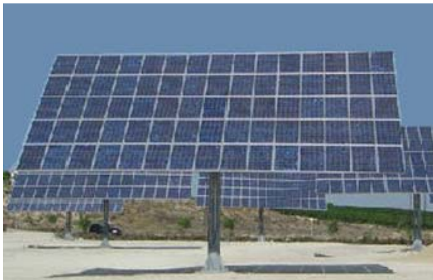
Figure 2.3: Illustration of a tracking photovoltaic panel
