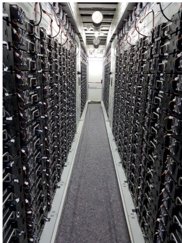
Figure 4.6: Li-Ion BESS internal design and implementation of a container used within a BESS. The image shows a series of sealed battery cell packs within a containerised module (Source: Enel Green Power)
