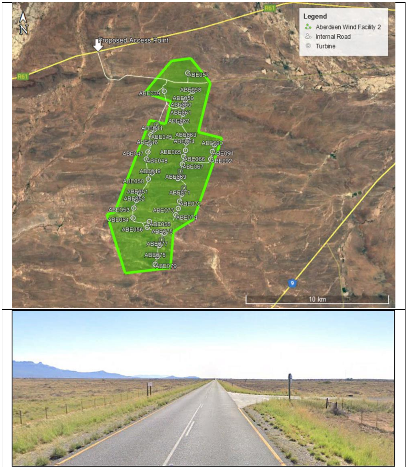
Figure 8.21: Map and photo of the existing gravel road providing direct access to the project site.
