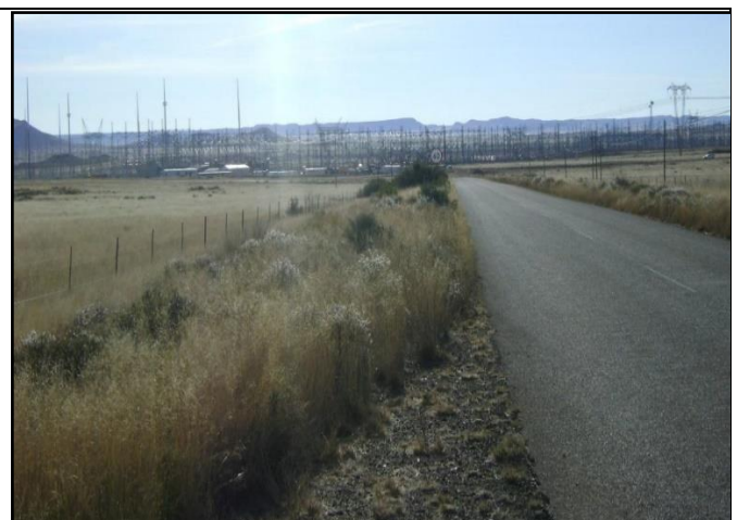
The Hydra Substation in the west of the study area.
