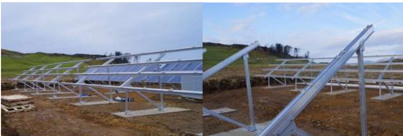
Figure 2.6: Frame structural details
