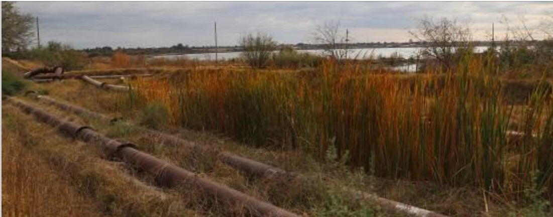
Modifications and severe degradation is evident along the shores of the Witpan.
