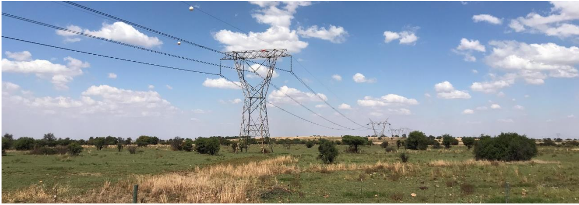
Figure 6.29: Photograph of some of the existing power lines in the study area
