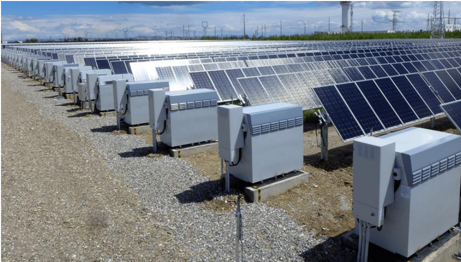
Figure 8.8 Example of battery storage units integrated as part of PV array (Source: nexttracker.com)
