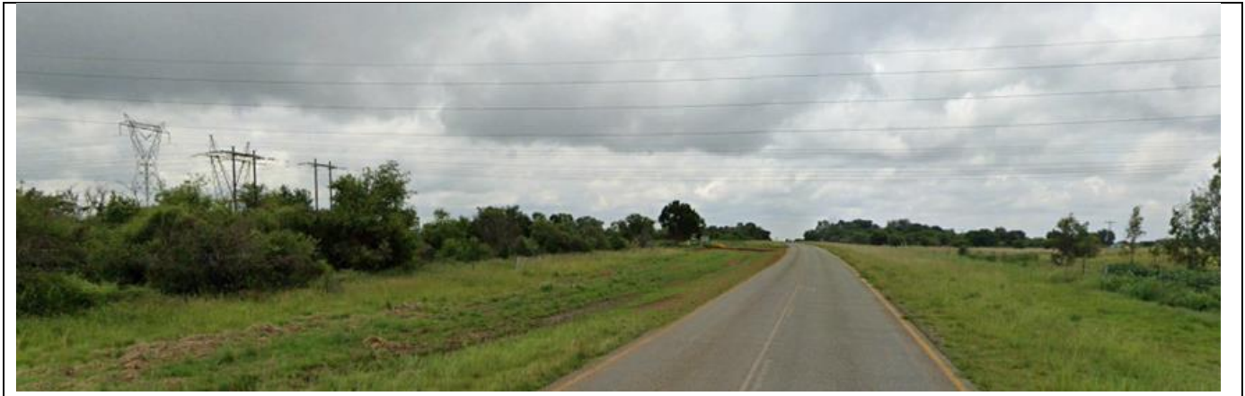
Figure 7.40 Power line infrastructure along the R505 arterial / main road
