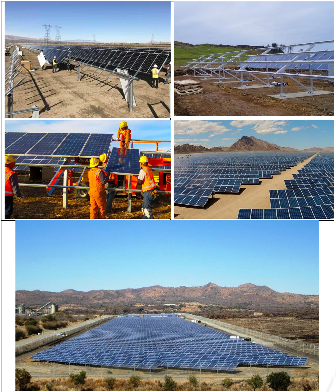
Figure 4.4: Photographs of the construction phase of a solar facility similar to those proposed
