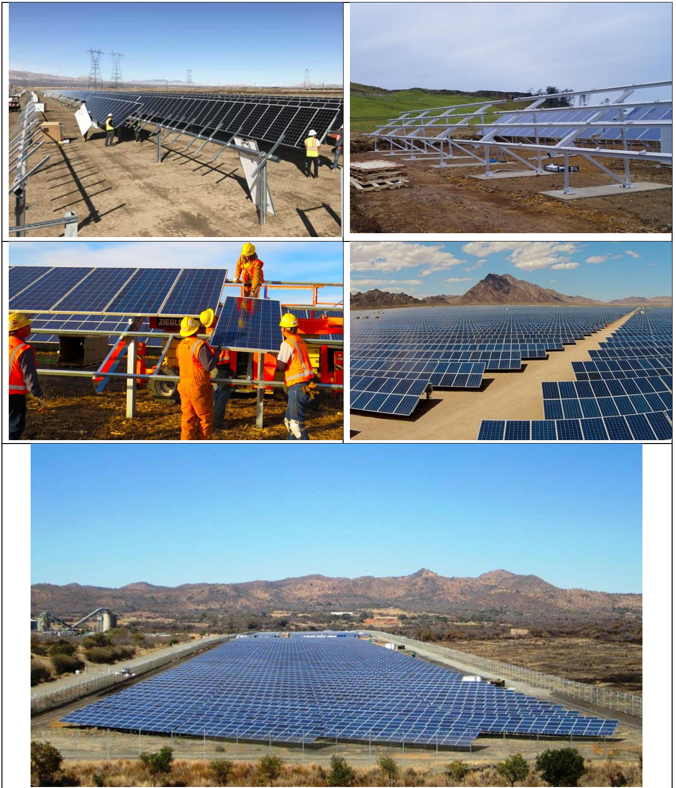
Figure 2.6: Photographs of the construction phase of a solar facility similar to those proposed (Source: https://medium.com/@solar.dao/how-to-build-pv-solar-plant-6c9f6a01020f ; https://www.shutterstock.com/video/clip-1028794-workers-mounting-panels-on-solar-power-plant-construction ; https://www.esi-africa.com/renewable-energy/kenya-construction-solar-farm-gets-green-light/ ).
