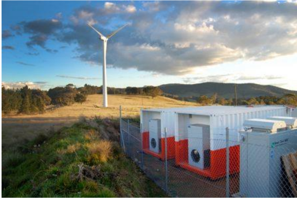
Figure 8.7 Example of battery storage units integrated as part of wind farm (Source: http://ultrabattery.com/applications/stationary-energy-storage/ )
