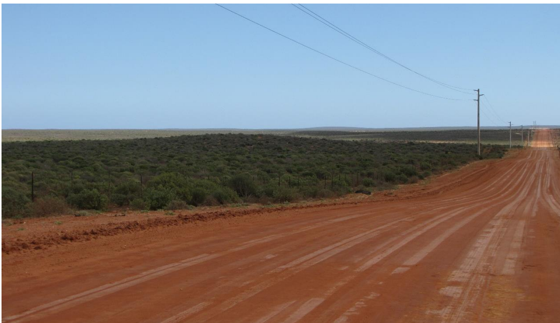
Figure 6.17: The Komaggas (east) to Kleinsee (west) road north of the proposed development site (to the left), as well as the 66kV overhead power line.
