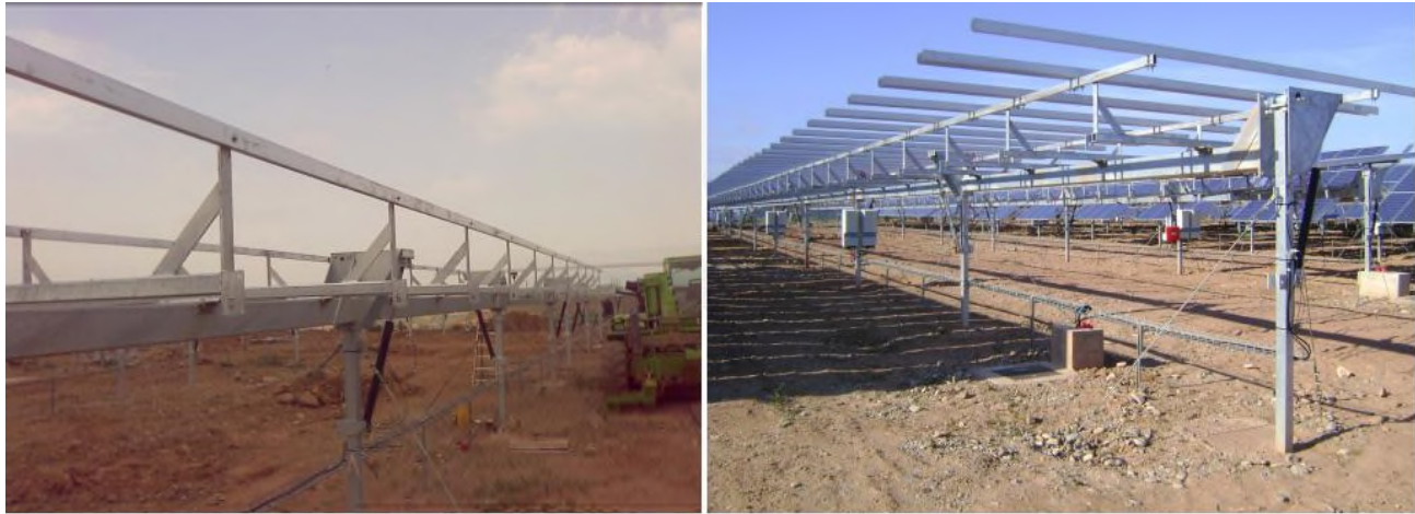
Figure 2.3: Frame, structural details (Photo courtesy of Igeteam, 2011).
