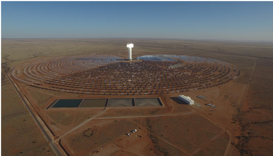
Figure 7.9: A view of the operational Khi Solar One located in the southern corner of Portion 3 of the Farm McTaggarts Camp No. 453 (source: www.energy.org.za ).
