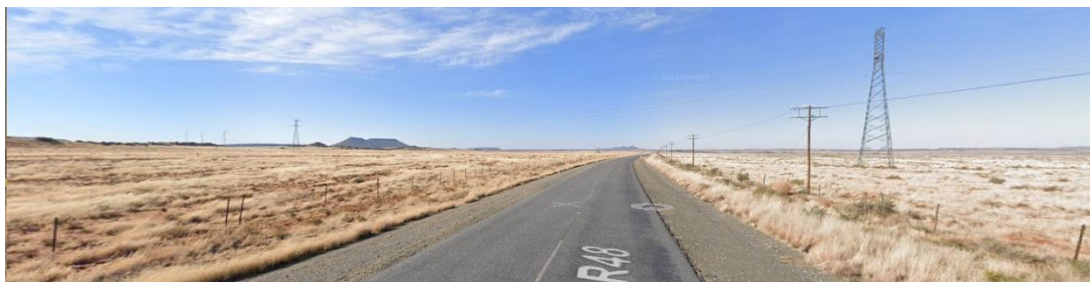
Figure 8.19: Powerline infrastructure within the study area (Photo: Google Earth)
