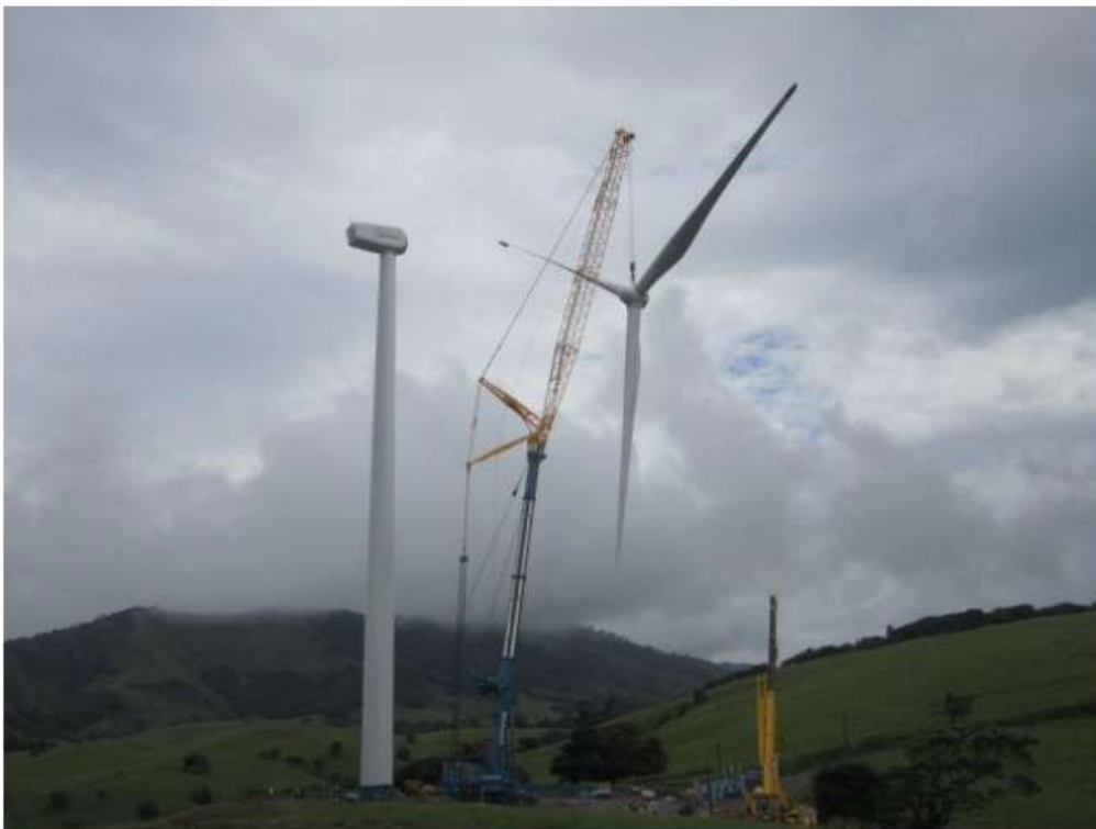
Figure 4.2: Example of a tower on which the blade is being mounted
