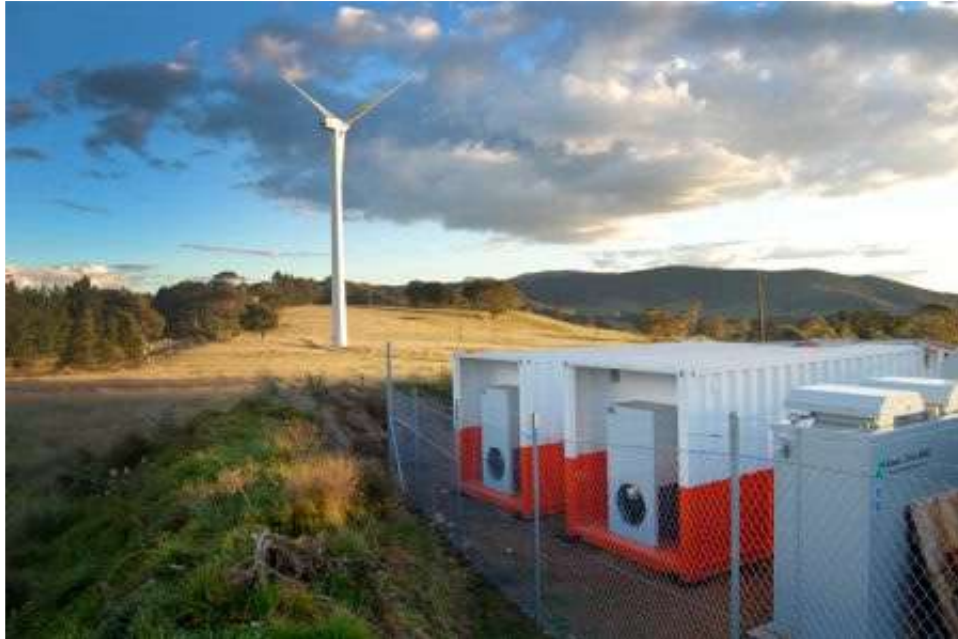
Figure 9.18: Example of battery storage units integrated as part of wind farm (Source: http://ultrabattery.com/applications/stationary-energy-storage/ )
