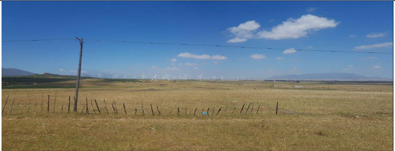
Photograph Simulation: From Point 5 - Road towards Saron - as per EA (110m hub height)
