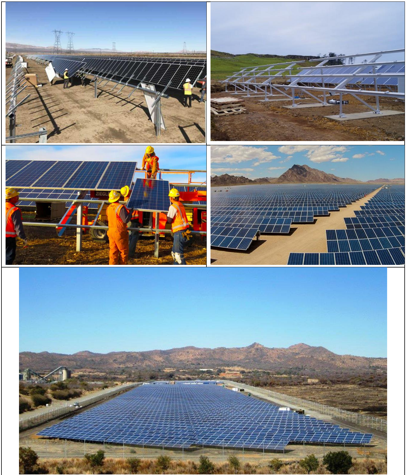
Figure 4.1: Photographs of the construction phase of a solar facility similar to those proposed
