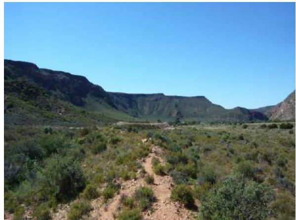
View east along the berm towards the dam
