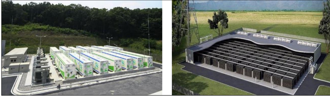
Figure 5-6. Battery Energy Storage Systems
