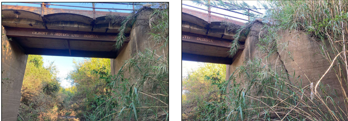
Figure 2: The existing bridge over the Ncandu River
