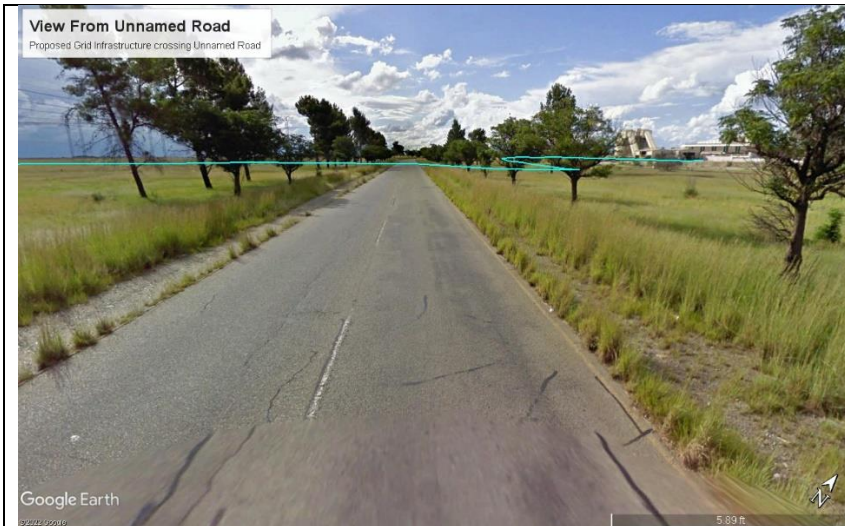
Figure 6.17. View of grid connection crossing from unknown road
