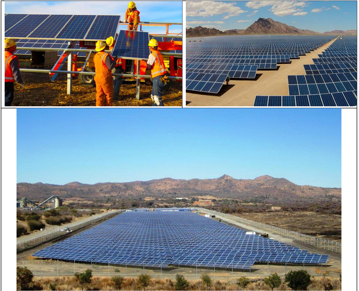
Figure 2.7: Photographs of the construction phase of a solar facility similar to the Harmony One Plant Solar PV Facility
