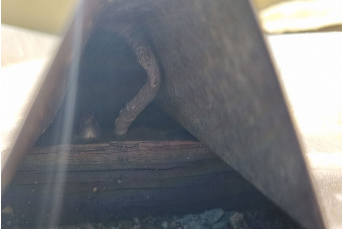
Figure 35: Image shows roof sheets has limited lifespan with visible previous repairs and damage to sheets. Replace fixing screws, fit poly closures to end of sheets.
