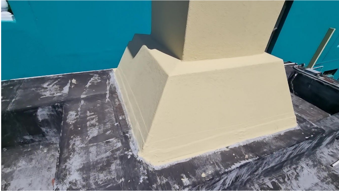
Figure 15: Image shows chimney wall waterproofing to be in good order.
