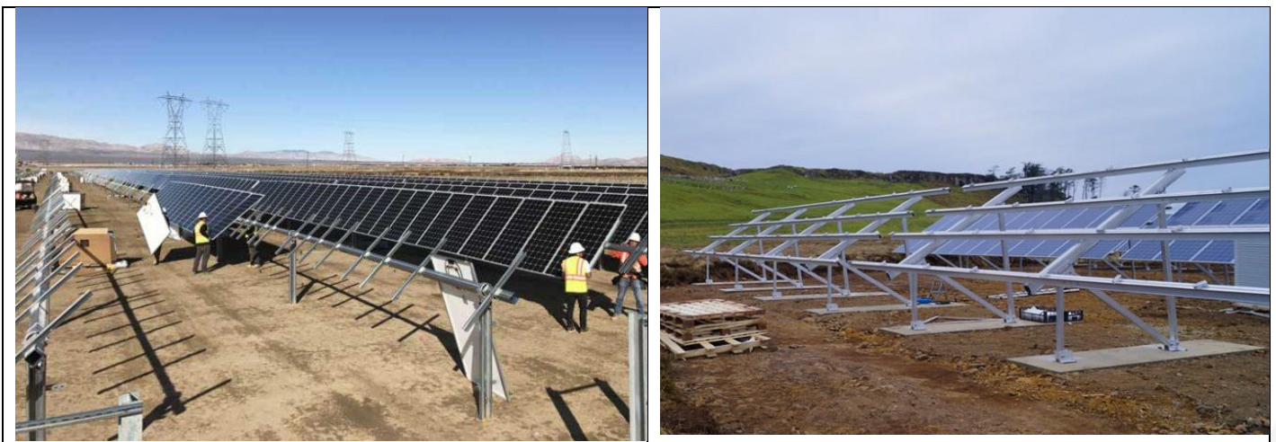
Figure 2.7: Photographs illustrating frame structural details
