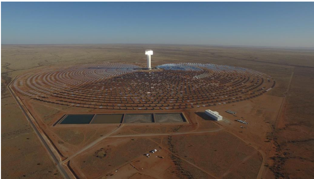
Figure 7.9: A view of the operational Khi Solar One located in the southern corner of Portion 3 of the Farm McTaggarts Camp No. 453 (source: www.energy.org.za ).
