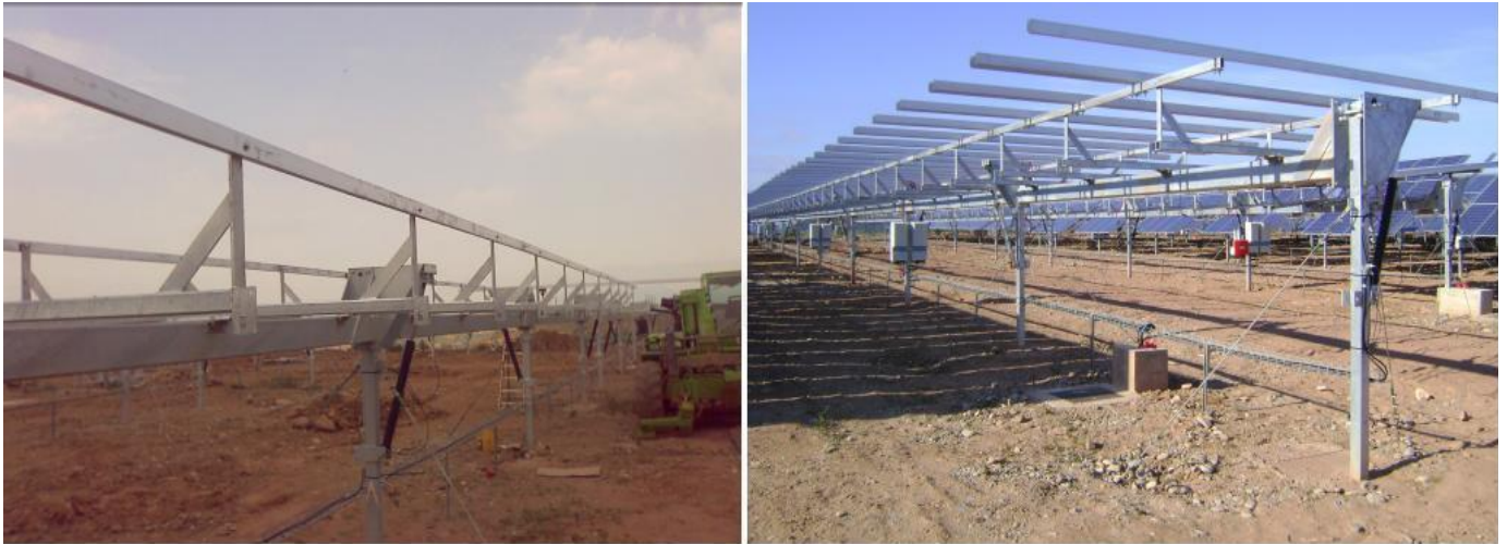
Figure 2.3: Frame, structural details (Photo courtesy of Igeteam, 2011).
