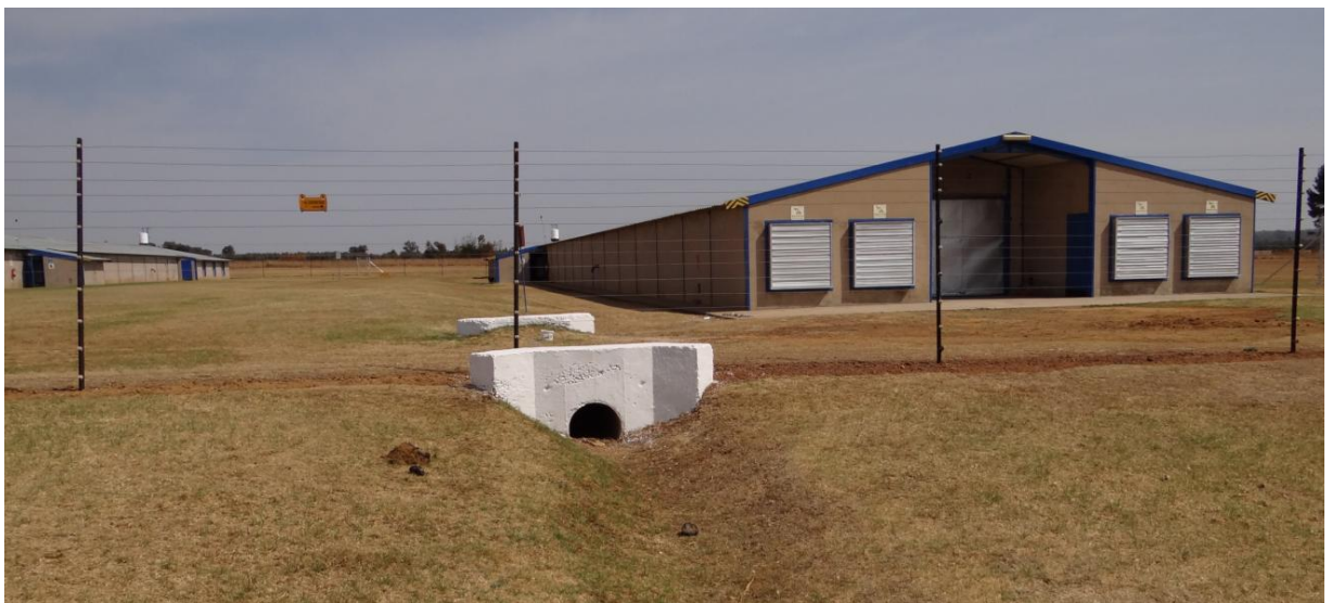
Photo 2: Existing facilities (broiler)
