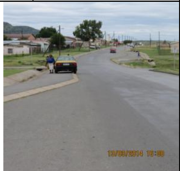
4. Road reserve through Steadville township south east of Ladysmith.
