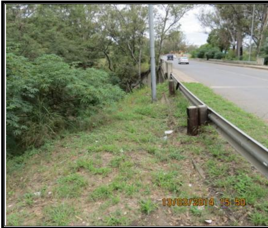
Photo 6: Watercourse Ladysmith (W6)
