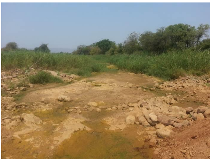
Figure 64: Upstream view of the GSP4 site on the Sand River showing the absence of water at this point.
