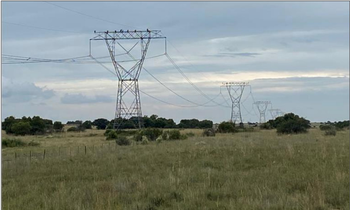
Figure 4-16: White-backed vultures roosting on the 400kV Hermes – Pluto 2 transmission line
