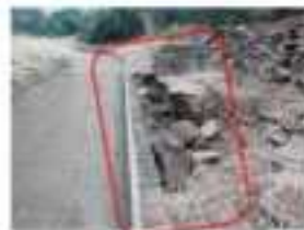
Figure 1: Photograph of the damage at Kloofendal as presented by FroK. This damage was caused by storm water overflow from the dam. Some trees should be cut before the spillway and then the dam.
