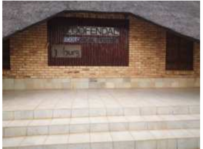
14. Entrance to the Ecological Centre
