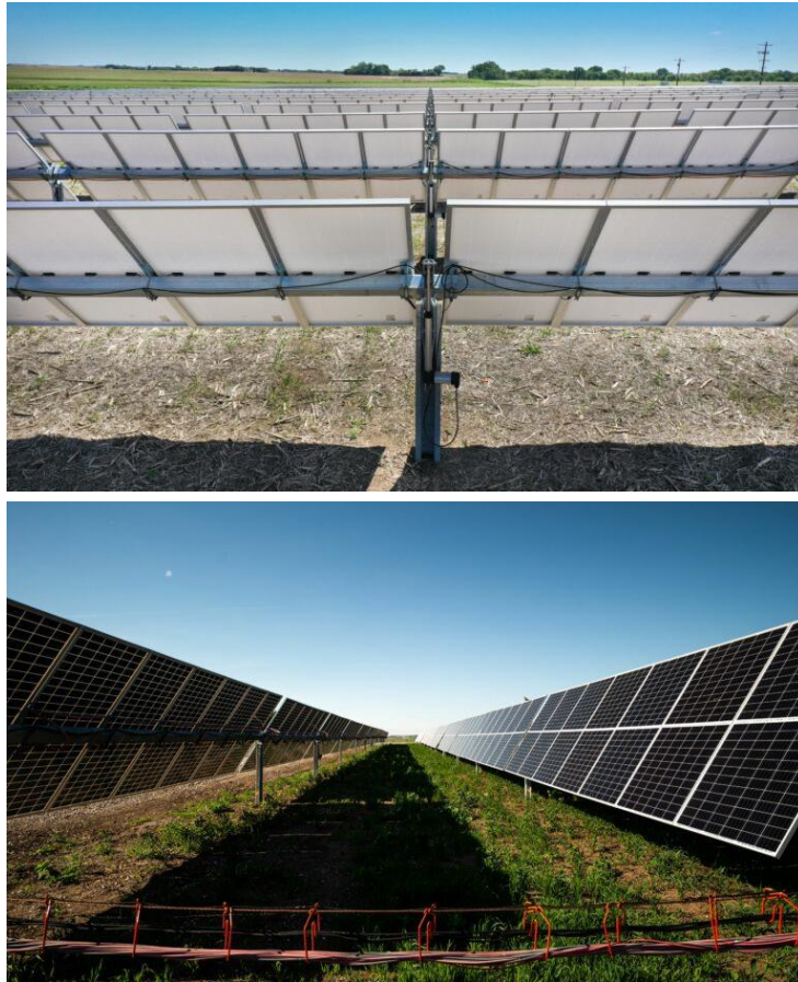
Figure 22: Monofacial (top) and bifacial (bottom) solar panels
