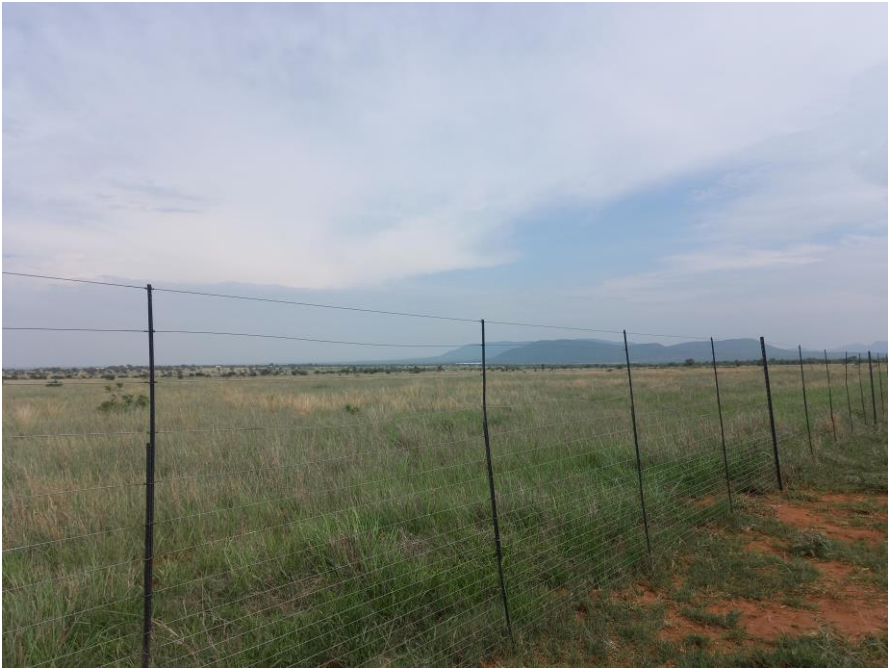
Figure 24: South eastern view of PV Site
