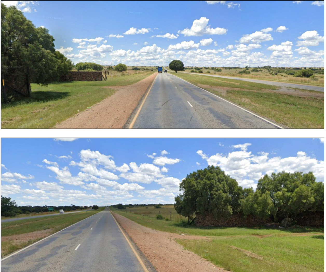
Figure 6-3: Sight distances at Access 1 to the east (top) and west (bottom)
