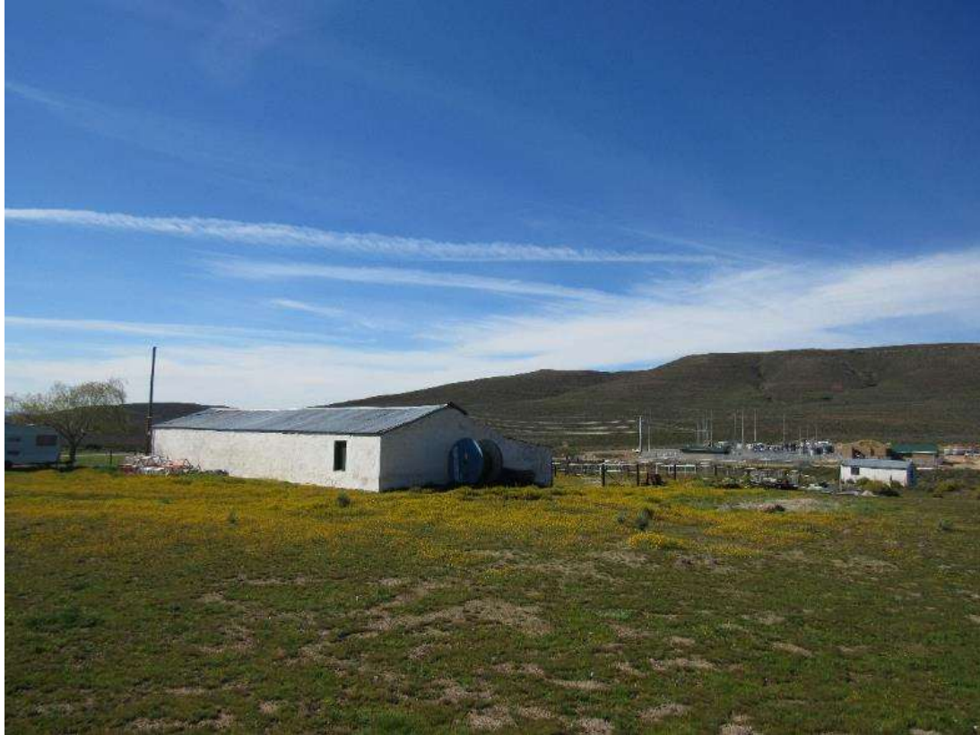
Figure 6-42: Bon Espirange Substation under construction
