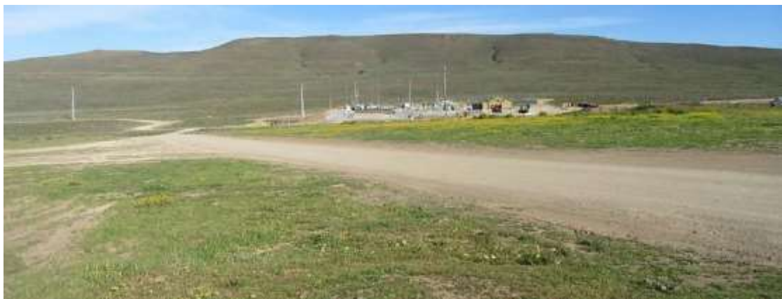
Figure 6-51: Roggeveld WEF substation on Bona Esperance viewed from near the farmstead located to the north-west
