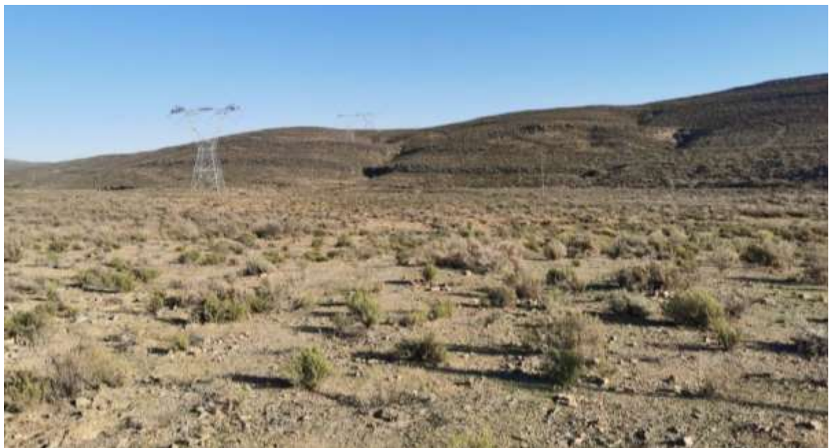
Figure 6-20: OHPL route near Komsberg substation
