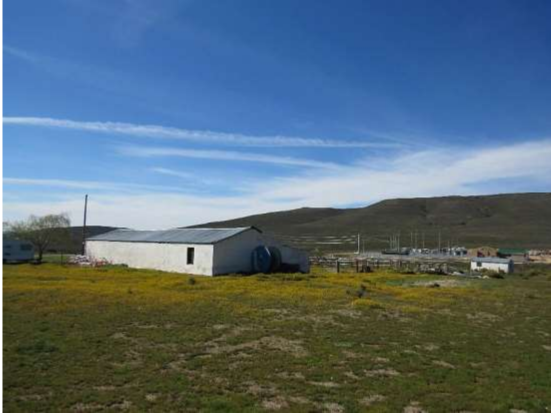
Figure 4-7: Bon Espirange substation under construction (source: SiVEST, 2021)
