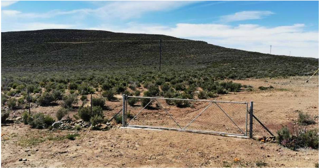
Figure 6-19: OHPL route east of R354 road towards Komsberg substation
