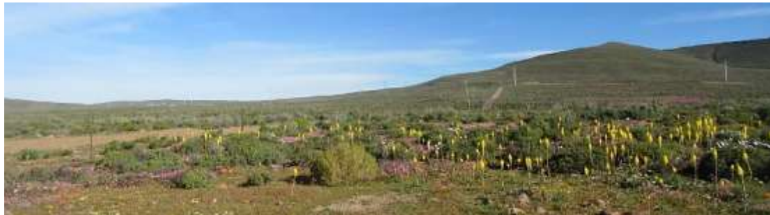
Figure 6-53: Newly constructed line from the Roggeveld WEF to Eskom Komsberg, seen from access road to Bona Esperance
