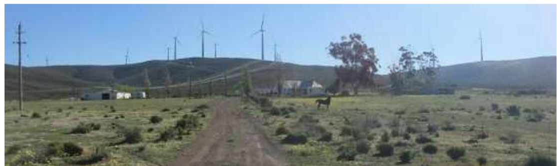
Figure 6-48: Farmstead and outbuildings on Bona Esperance seen from entrance road. Note the turbines (Roggeveld WEF) and overhead lines feeding into Bon Espirange substation. The impact is contained to the west and south of the farmstead
