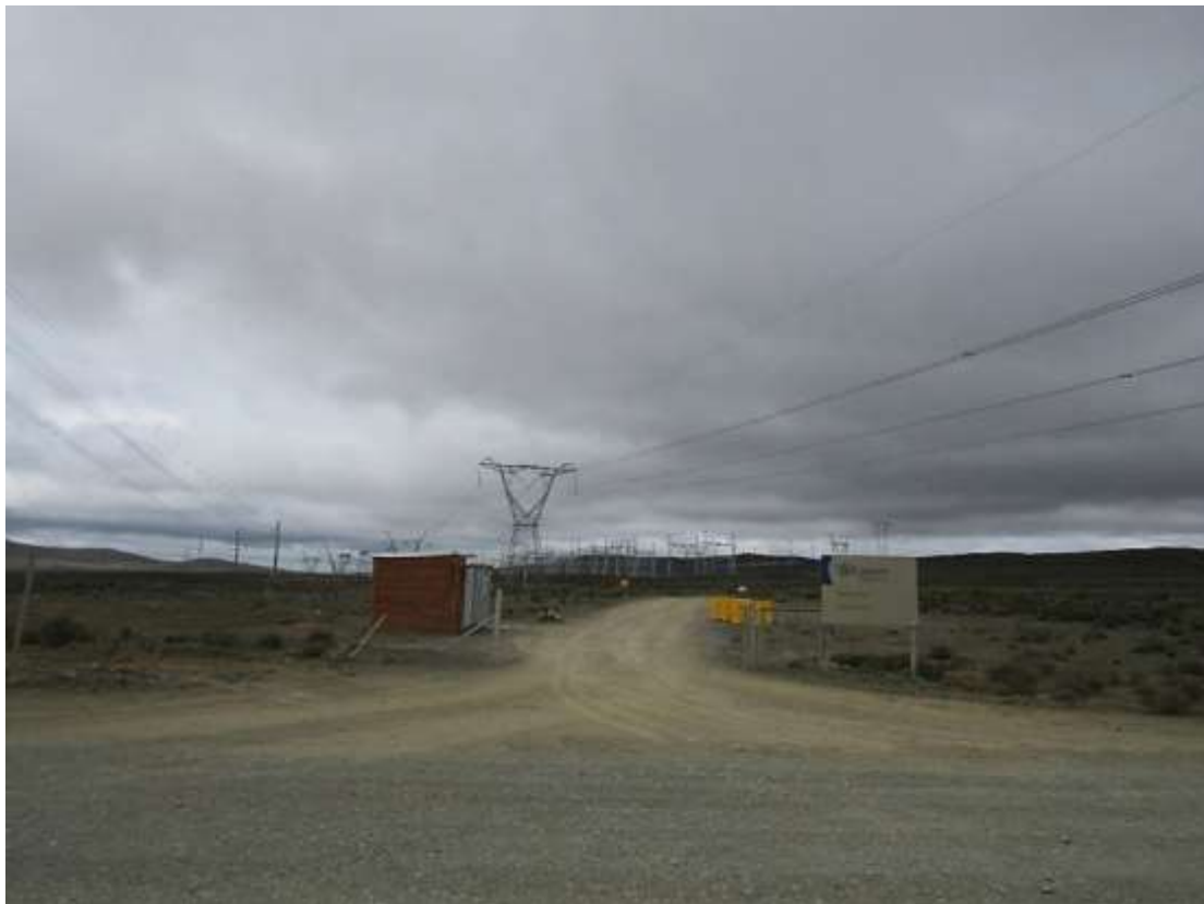
Figure 4-8: Komsberg substation (source: SiVEST, 2021)
