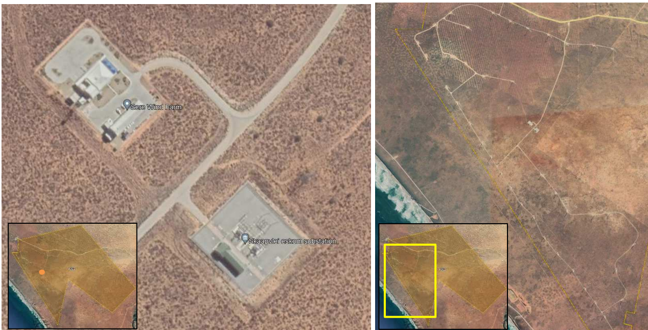
Figure 38: Existing Wind Farm O&M Buildings and Skaapvlei Substation (left); Wind Turbines and access roads (right)
