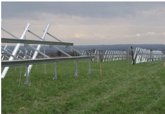
Figure 5: Installation of panel mounting structures
