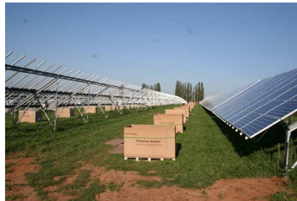
Figure 6: Placing panels onto support structures
