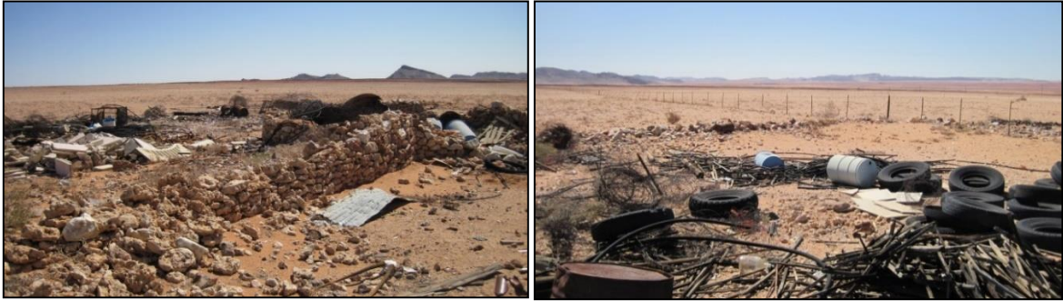
Figure 6-35: An older disused kraal made from clacrete blocks also serving as a farm dump.
