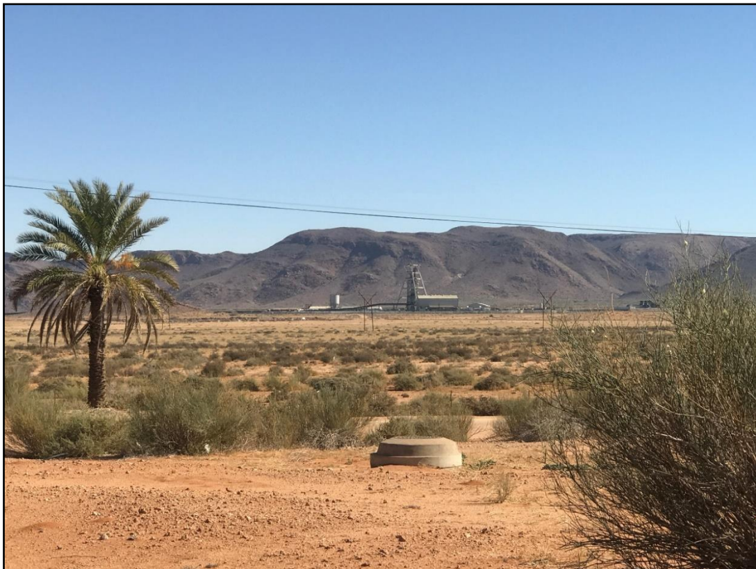
Figure 6-41: Mining operations at the BMM mine with Aggeneys Mountain in the background.
