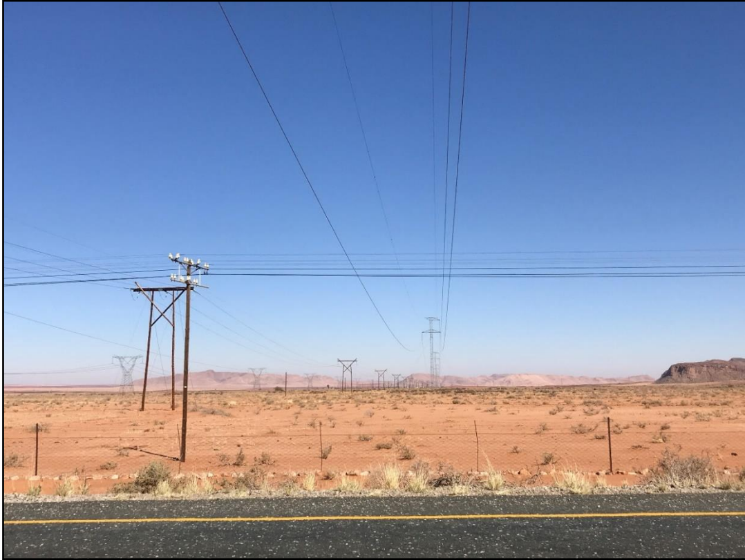
Figure 6-40: Power lines crossing the access road to Aggeneys near the N14.
