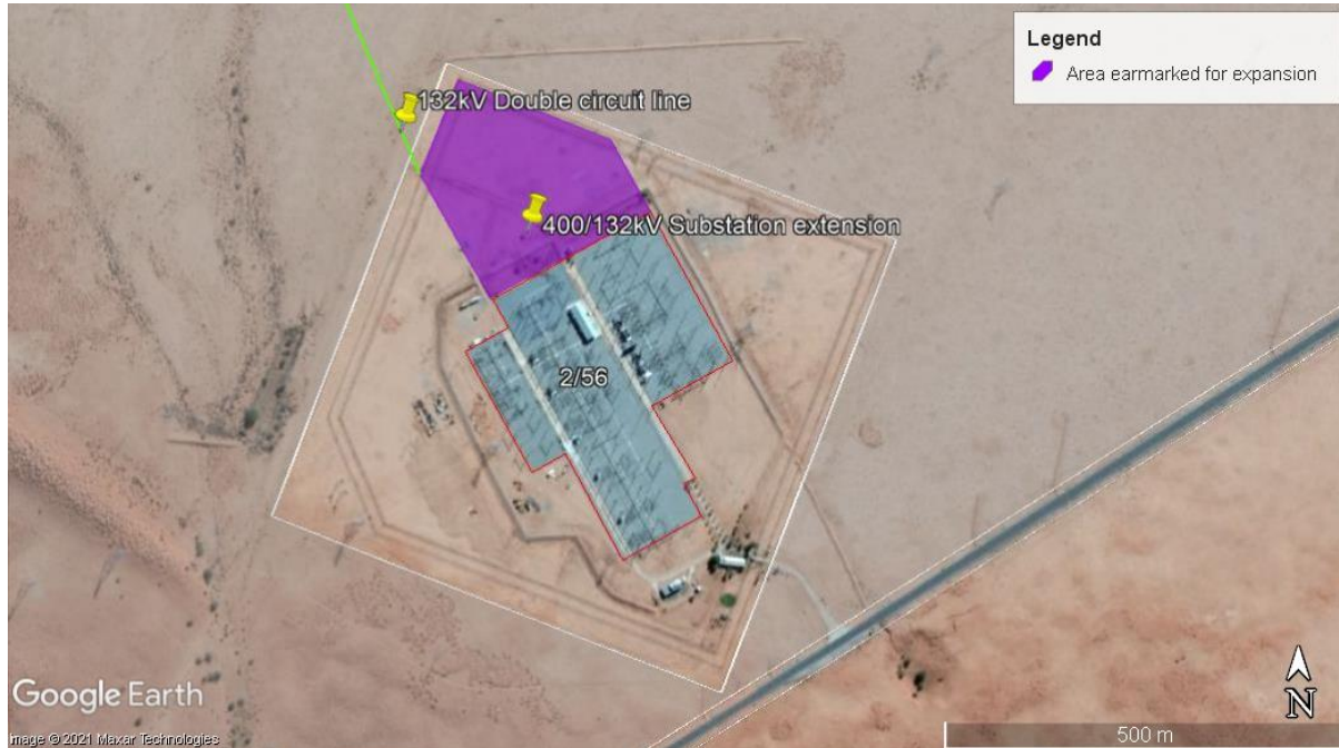
Figure 4-6: Area earmarked for the expansion of the Aggeneis substation
