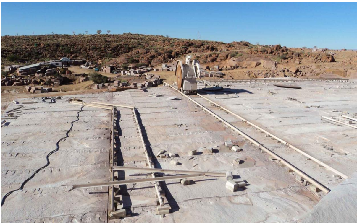
Photo 2 Circular saw with tracks being laid
