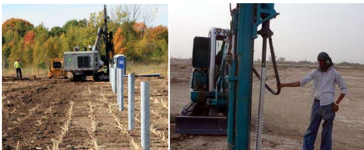
Figure 3: Driven/ Rammed Steel Pile (left) and Ground Screw (right) are the preferred mounting technology (Aristida PV, 2022)
