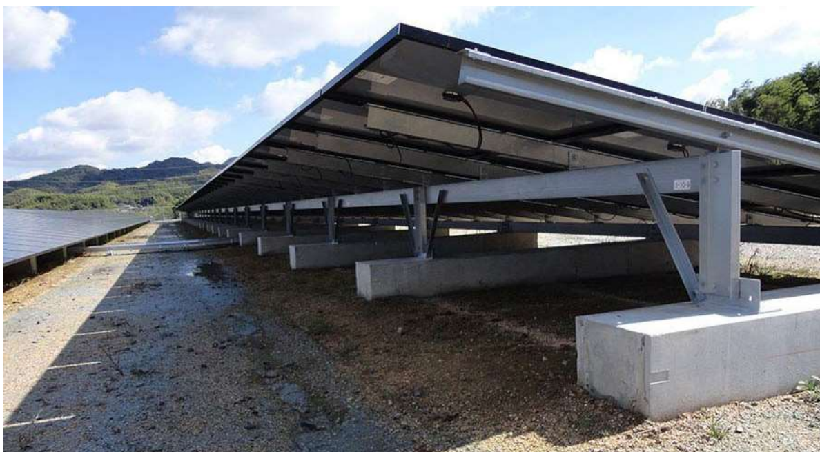
Figure 2: Cast Concrete Foundation - alternative mounting (Aristida PV, 2022)
