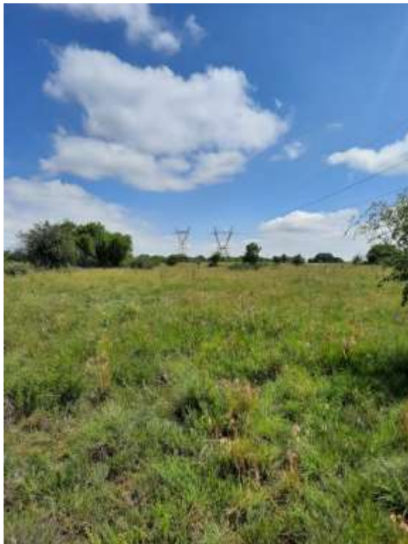
Figure 19: Existing powerlines traversing the Aristida PV site.(van der Walt, 2022).
