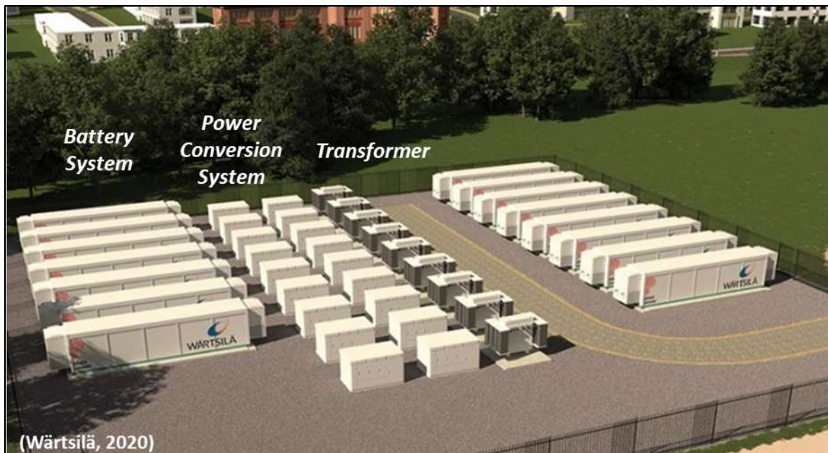
Figure 6: Pivot Power's proposed 50MW lithium-ion battery in Kemsley, Kent.
