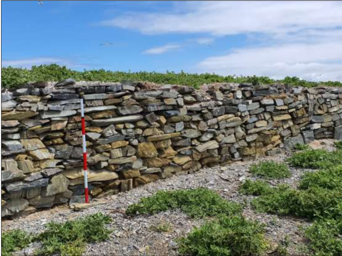
Wall 2bcd (b= right side, d= left side).
