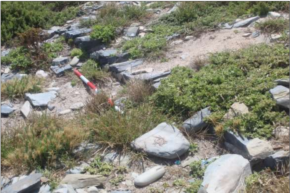
Wall 13, revetment wall, may be partially buried.
