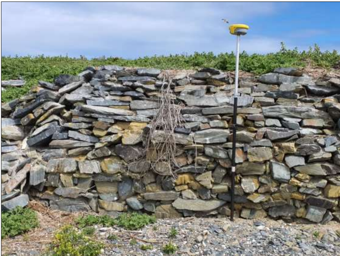
Wall 2g (west of Wall 2f).
