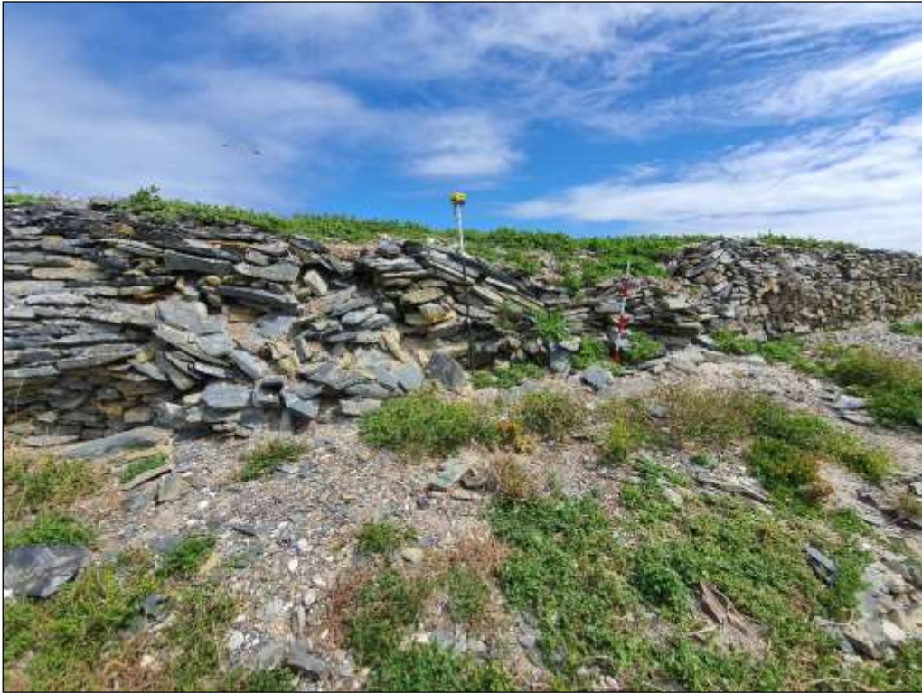
Wall 3, partially collapsed section (west of Wall 2).
