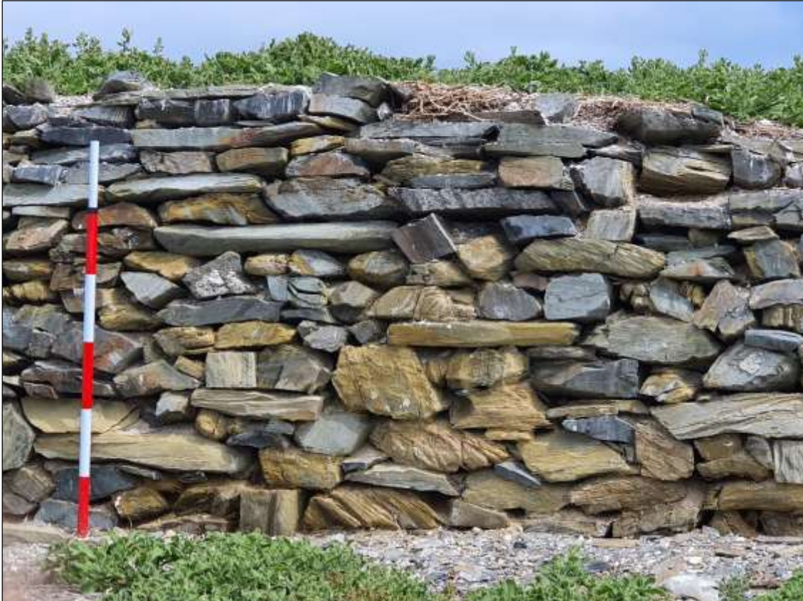
Wall 2e (west of Wall 2d).
