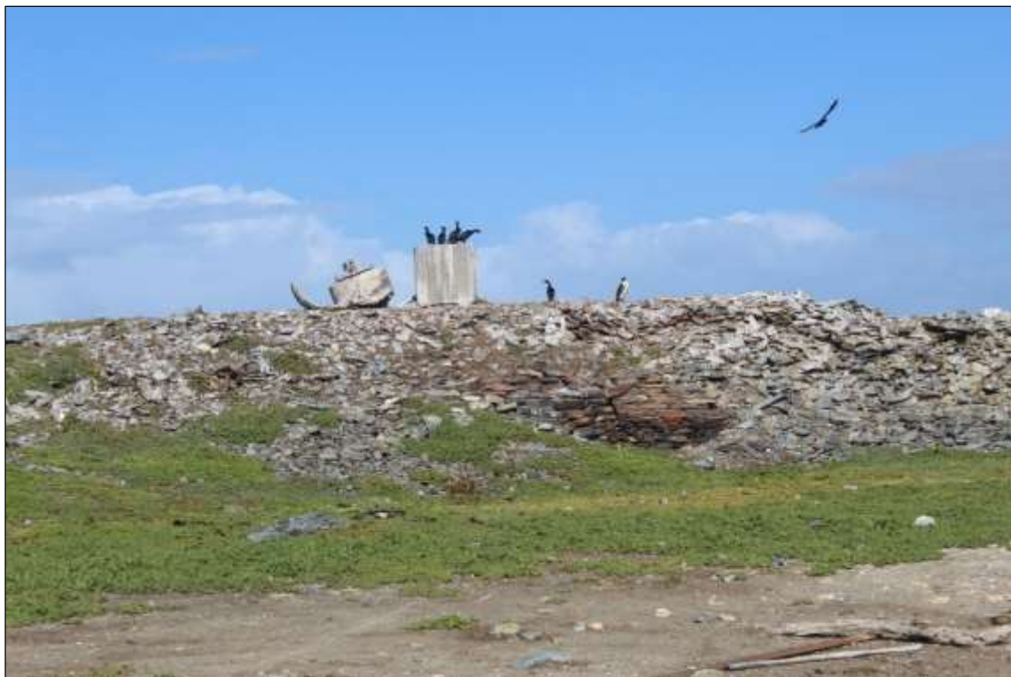
Wall 19, wide view shows collapses on both sides.
