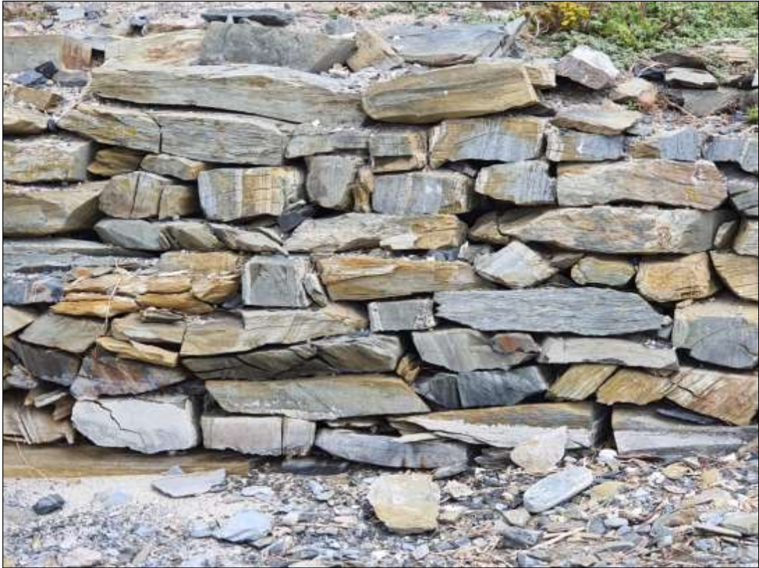
Wall 8, midsection, close-up view.
