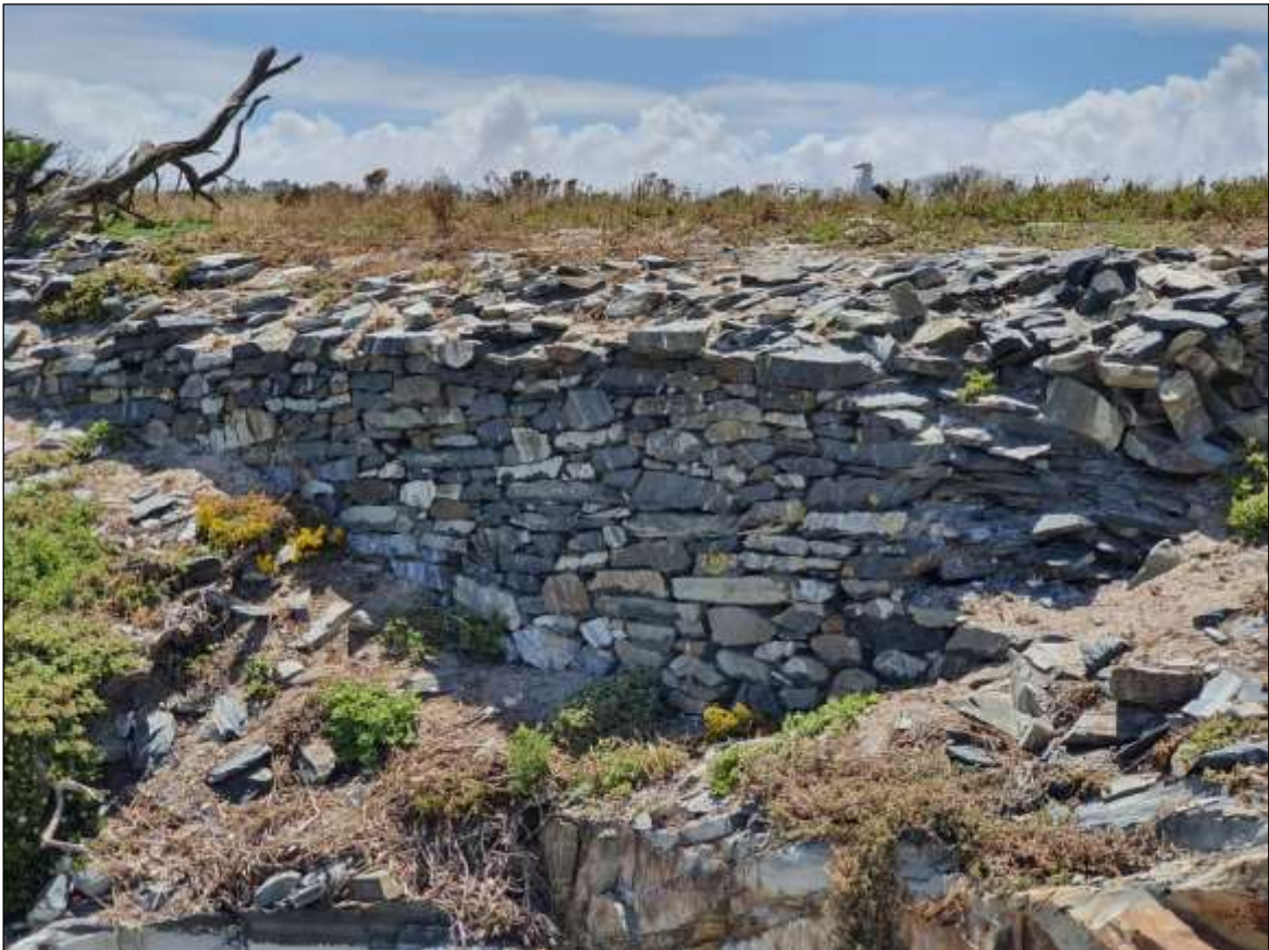
Wall 15, revetment wall, fairly well preserved.
