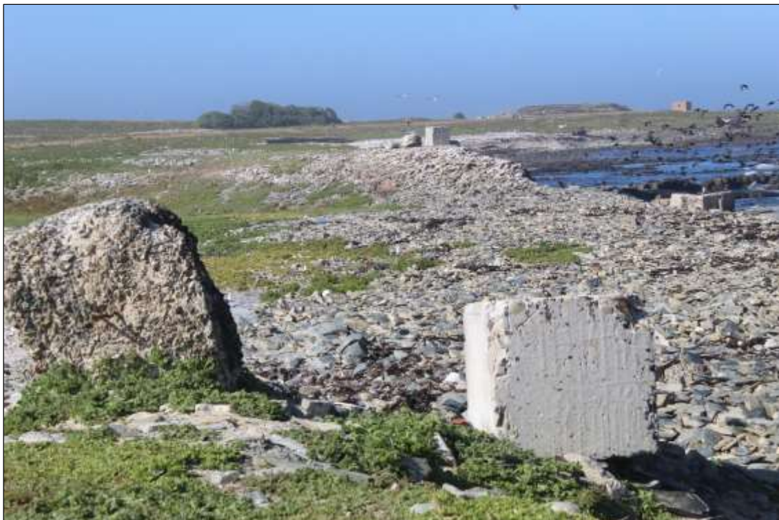
Collapsed mid-section of main wall, view from the north.
