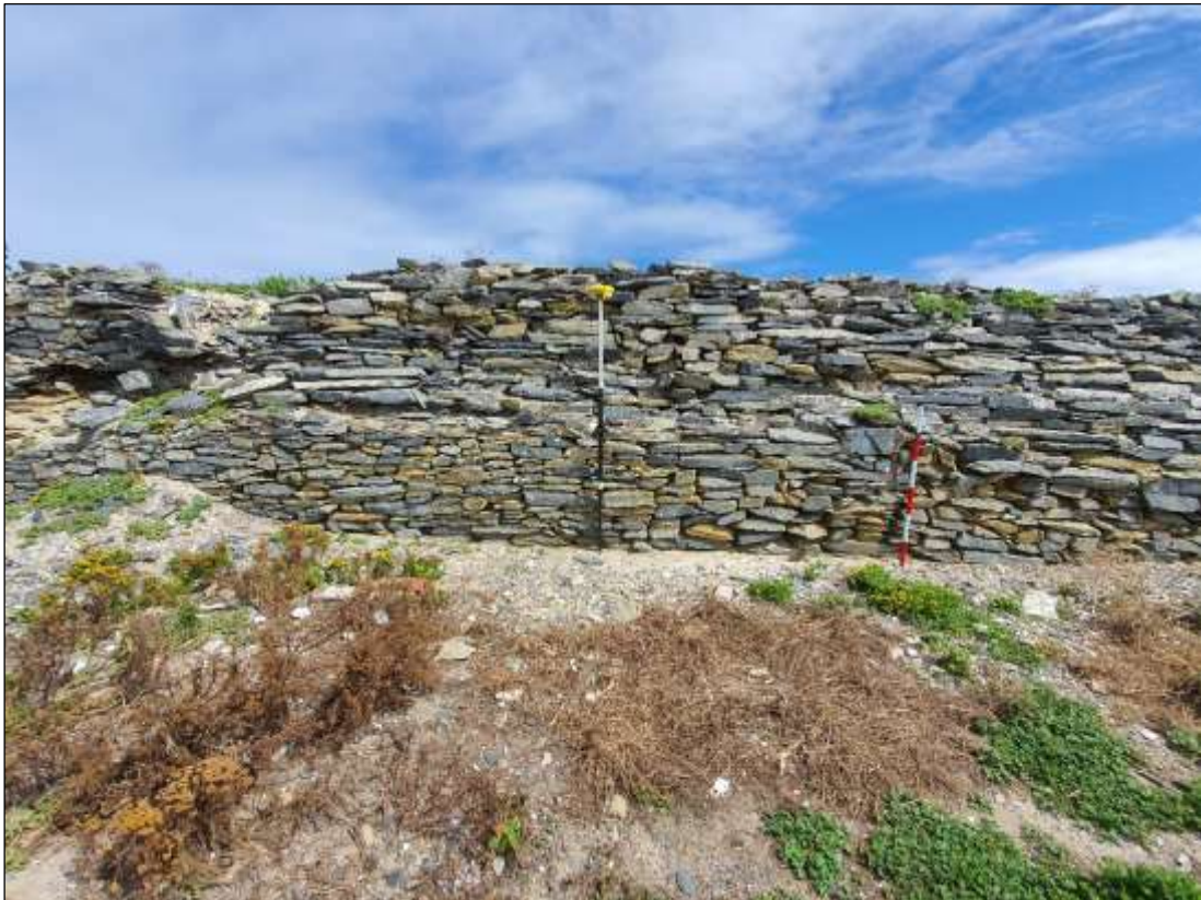
Wall 3b (west of 3a).
