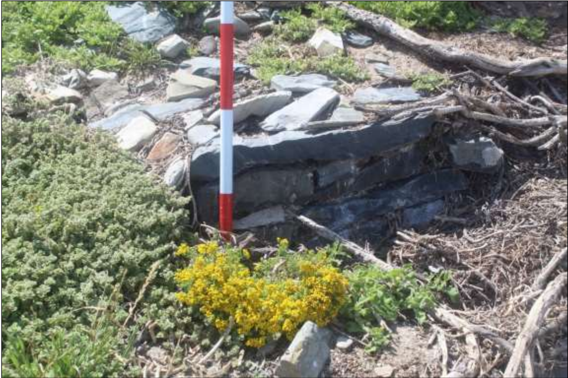
Wall 14, revetment wall.
