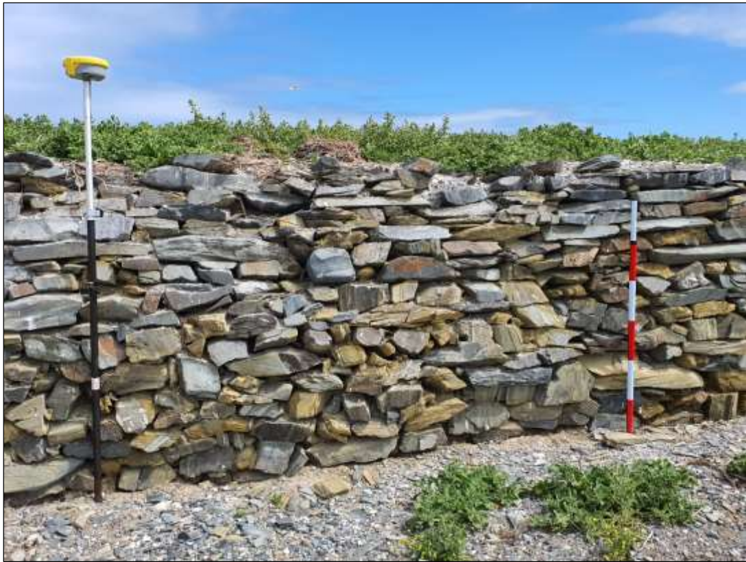
Wall 2f (west of wall 2e).
