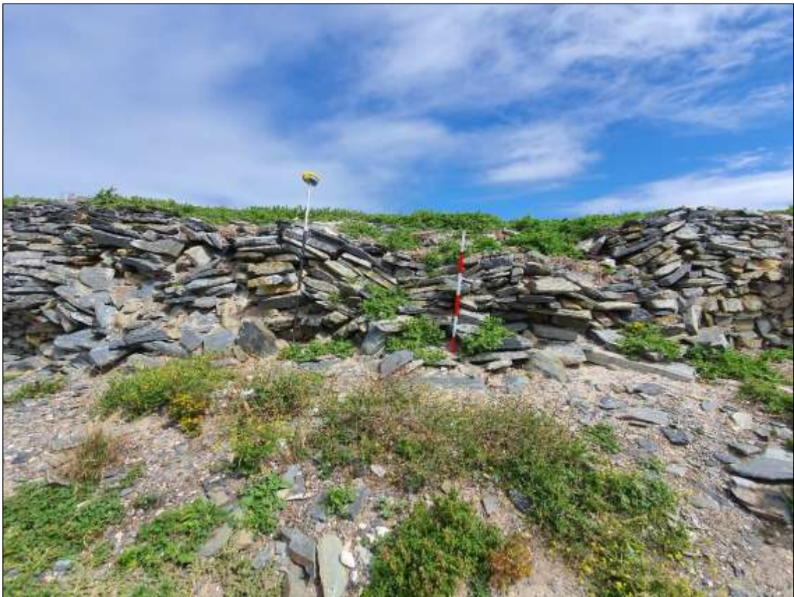
Wall 3, closer view.
