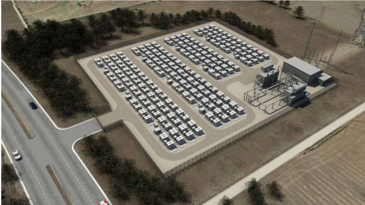
Figure 14: SolarCity's Tesla Battery Storage Facility, Hawaii (AMDA Developments, 2022)
