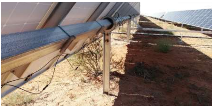
Figure 6: Completed ramming and assembly showing vegetation remaining intact beneath the modules.
