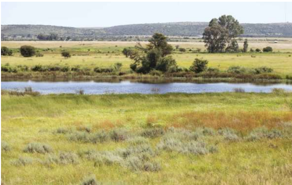
Figure 49: In-channel dam (Dam 1) at the northwestern part of the site. Areas in the background are outside the site. (Terblanche, 2022)
