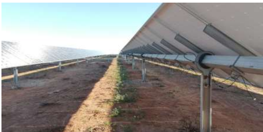
Figure 7: Showing vegetation re-establishing along the driplines of the arrays within weeks after installation.
