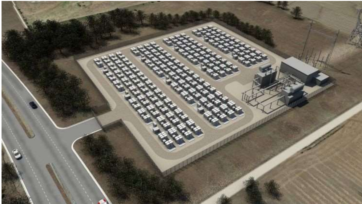
Figure 13: SolarCity’s Tesla Battery Storage Facility, Hawaii (AMDA Developments, 2022)
