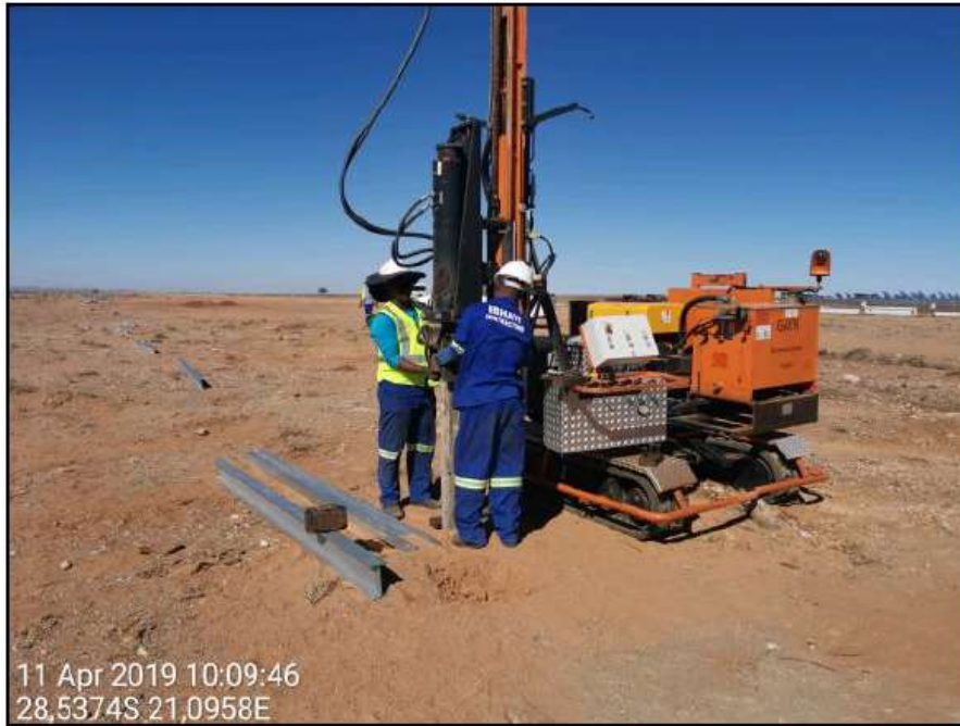
Figure 5: Ramming of steel piles into the pre-drilled / backfilled holes.
