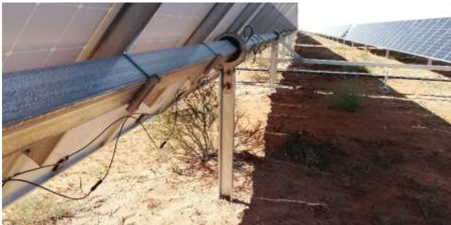
Figure 7: Completed ramming and assembly showing vegetation remaining intact beneath the modules.
