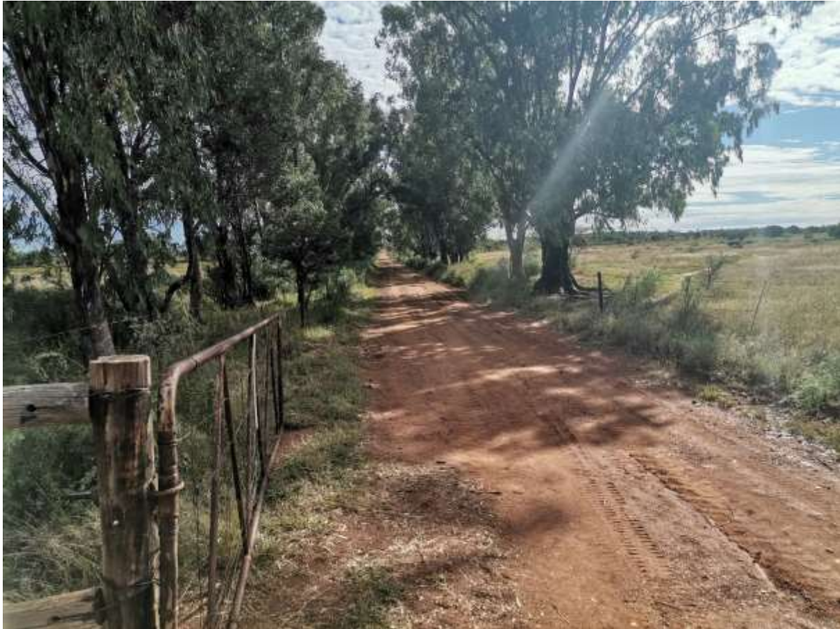
Figure 22: Existing farm access road that will be utilised to access Doornhoek 2 PV.
